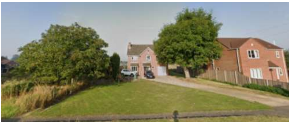
Street view of 29 Wisbech Road. (Google Earth 2022).
