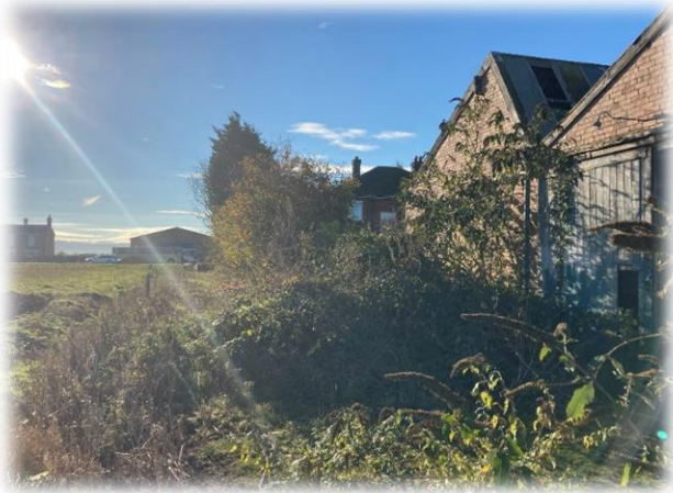
View of existing buildings.
