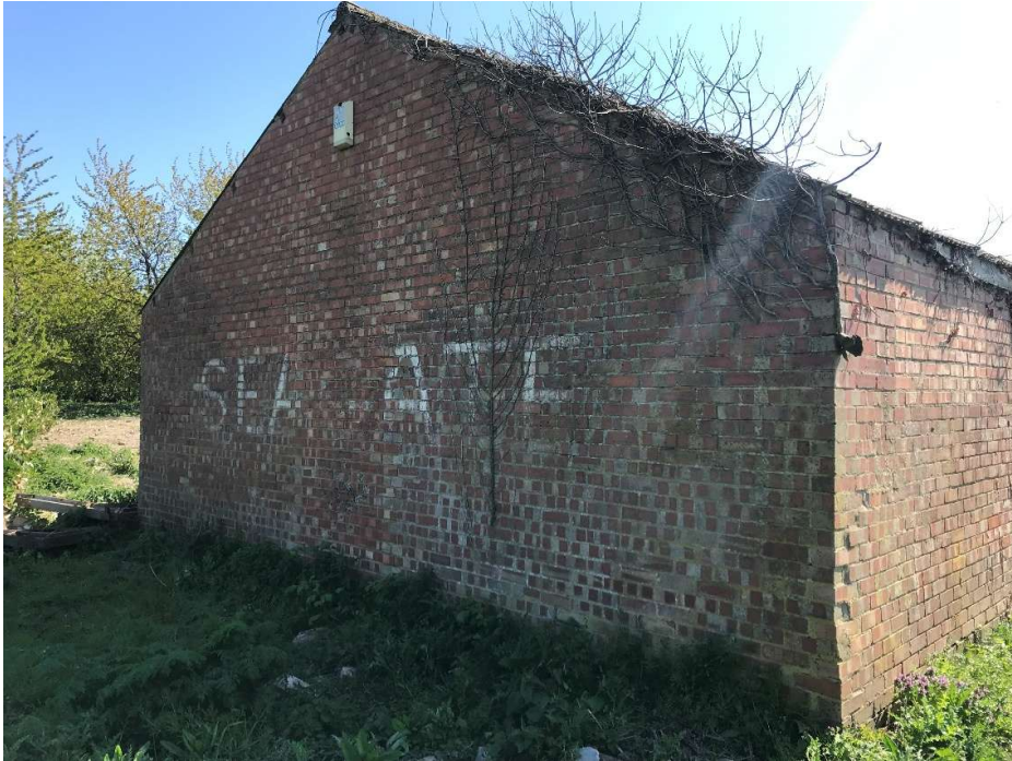
Photo 5. Nothern Gable End Elevation
