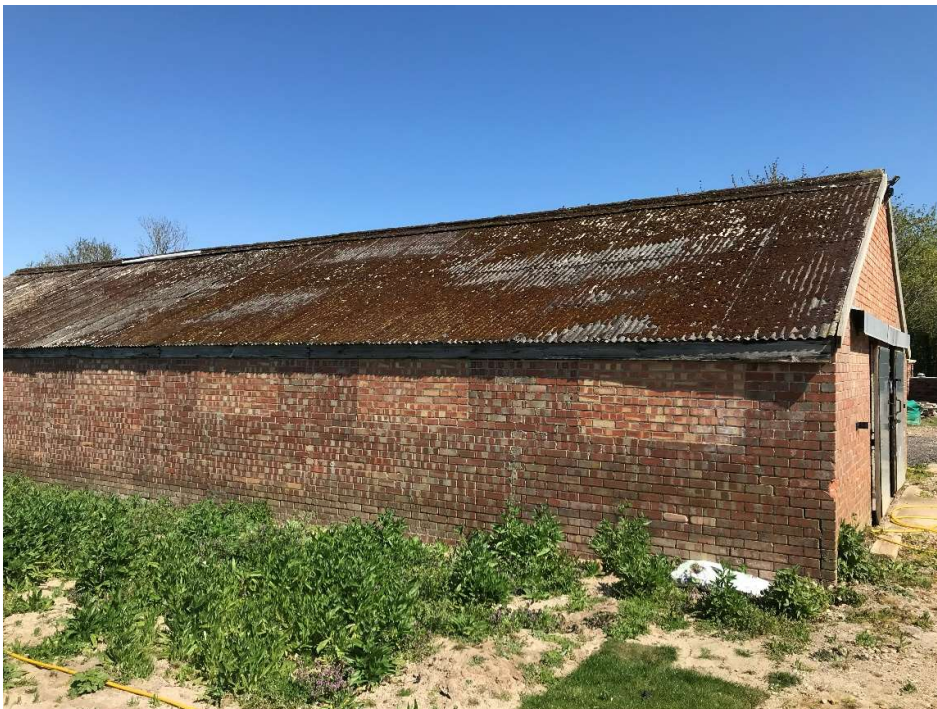
Photo 4. West Side Elevation – southern end
