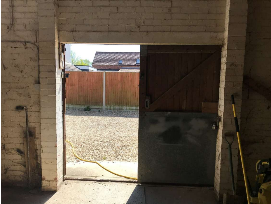
Photo 9. Front Door on Southern Gable End Elevation take from inside. PC Lintel above door
