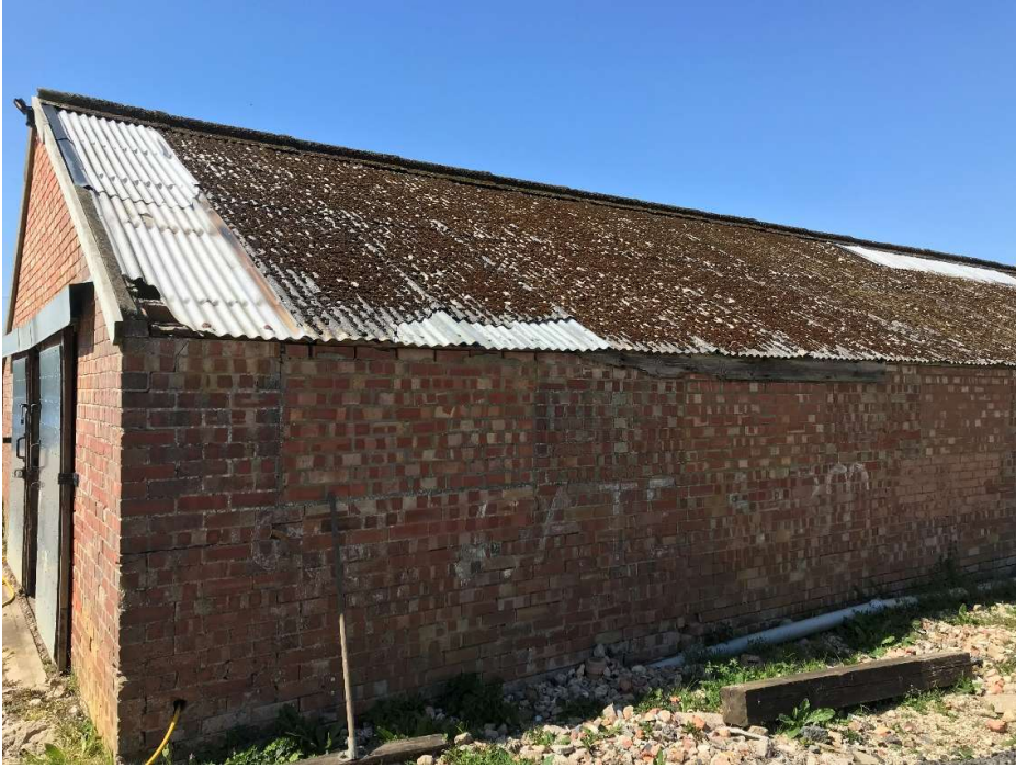
Photo 1. East Side Elevation – southern end
