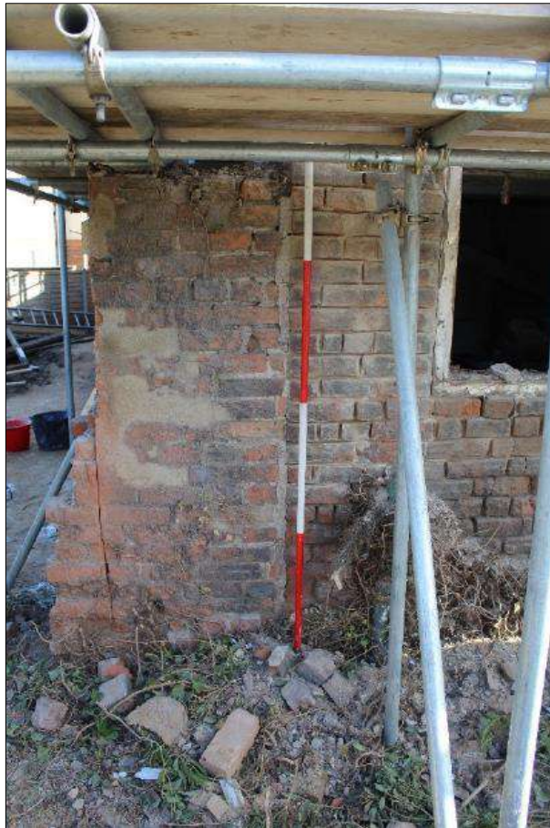
Plate 7 (shot 16): Straight joint between former extension and the stable. Looking east-northeast, 2m scale
