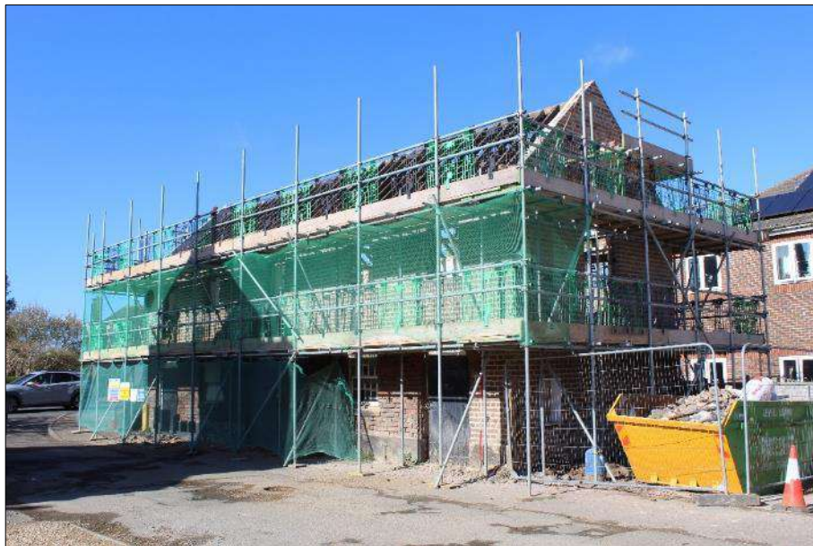
Plate 1 (shot 1): General view of stable and coach house, looking west-northwest, 2m scale
