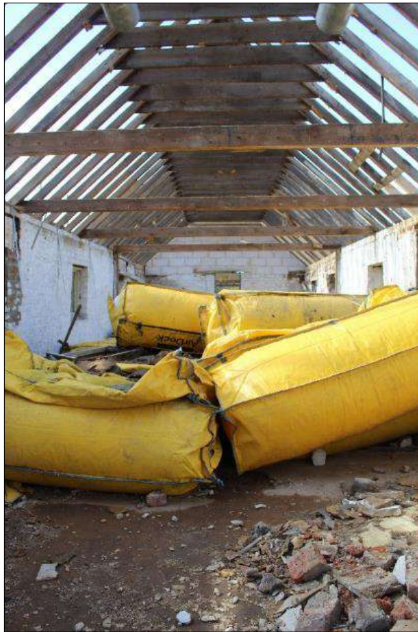
Plate 19 (shot 54): General view of the loft. Looking west-southwest
