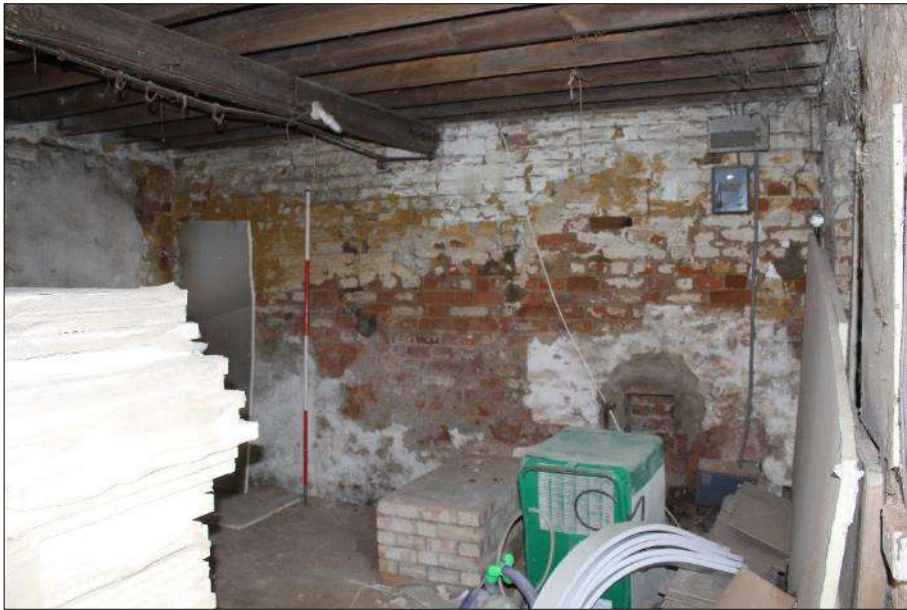
Plate 12 (shot 28): General view of the ground floor, looking northeast, 2m scale
