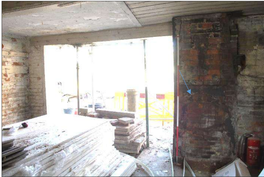
Plate 14 (shot 33): Blocked up fireplace on the northwest wall. Arrow points to segmental arch. Looking west-northwest, 2m scale
