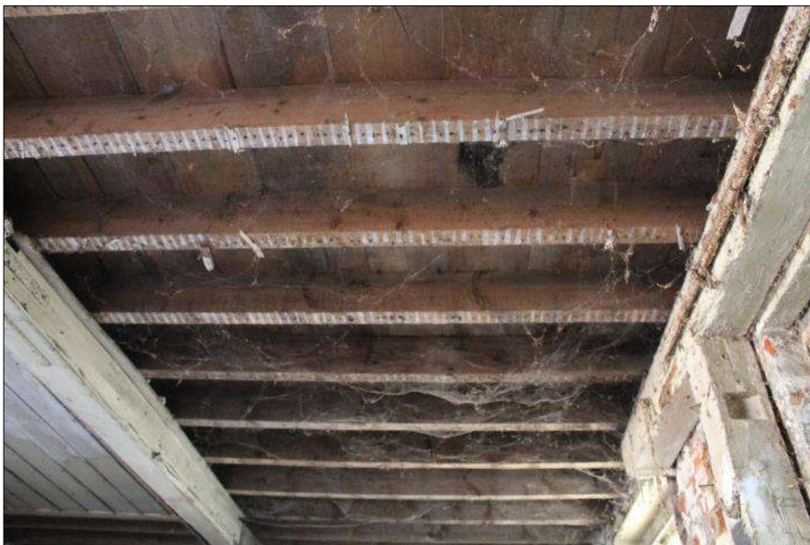
Plate 13 (shot 34): Loft floor planks and joists. The latter showing traces of former laths from a removed plastered ceiling. Looking east-northeast
