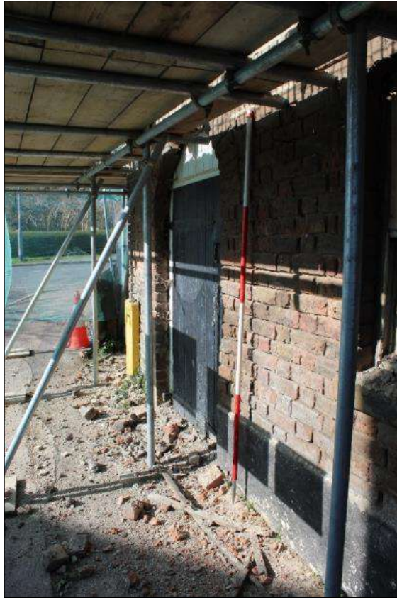
Plate 2 (shot 7): Representative shot of doorway. Looking west, 2m scale
