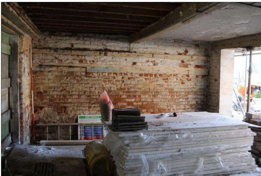
Plate 11 (shot 26): General view of the ground floor, looking west-southwest, 2m scale
