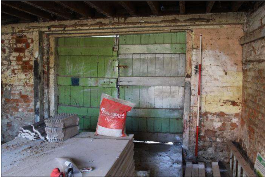
Plate 10 (shot 25): Plank and batten double coach doors. Looking south-southeast, 2m scale
