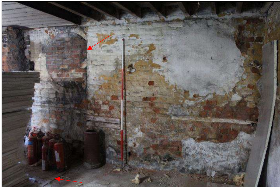
Plate 15 (shot 30): Bricked up portholes on the northwest wall, arrows point to area of former partition or fixture. Looking west-northwest, 2m scale
