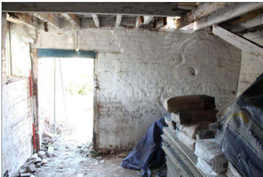
Plate 18 (shot 45): General view of southwest room showing bricked up porthole window. Looking north-northwest, 2m scale
