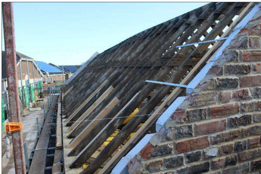
Plate 8 (shot 67): Repaired roof structure, looking east-northeast
