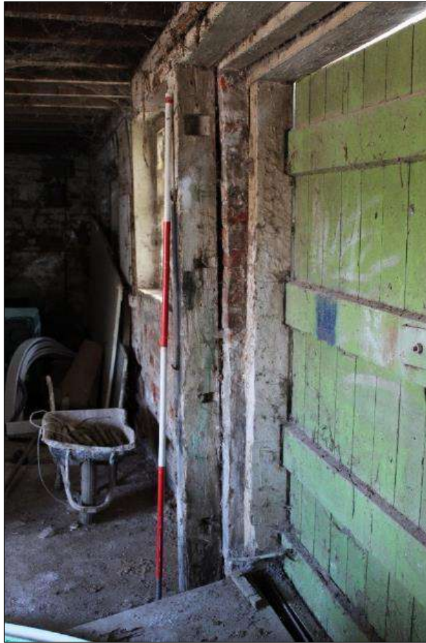
Plate 16 (shot 35): Post (reused timber) with empty mortices. Looking east-northeast, 2m scale
