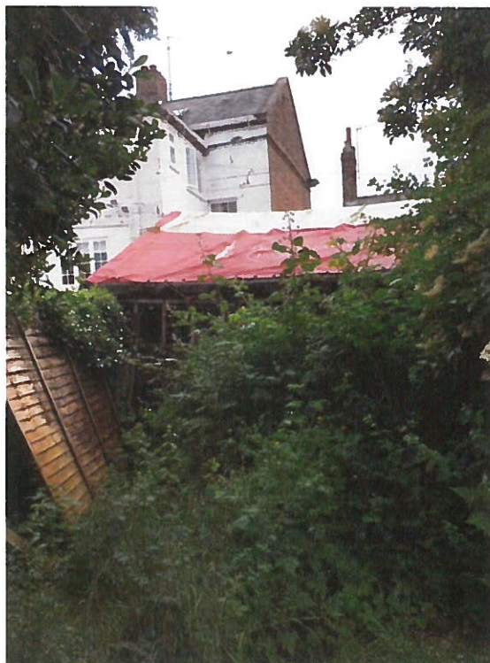
Wooden garage to be demolished
