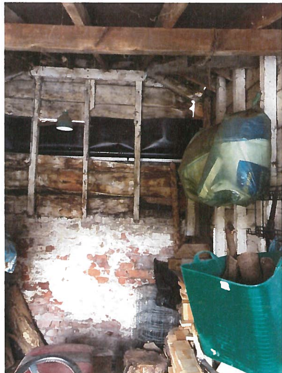
Photograph of the interior of the brick outbuilding to be rebuilt
