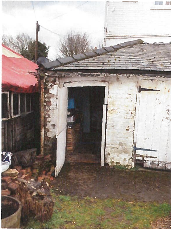
Photograph of the left-hand side (north west elevation) of the brick outbuilding to be rebuilt
