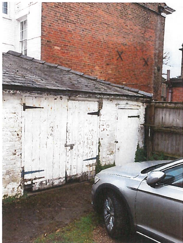
Photograph of the right-hand (north west elevation) side of the brick outbuilding to be rebuilt
