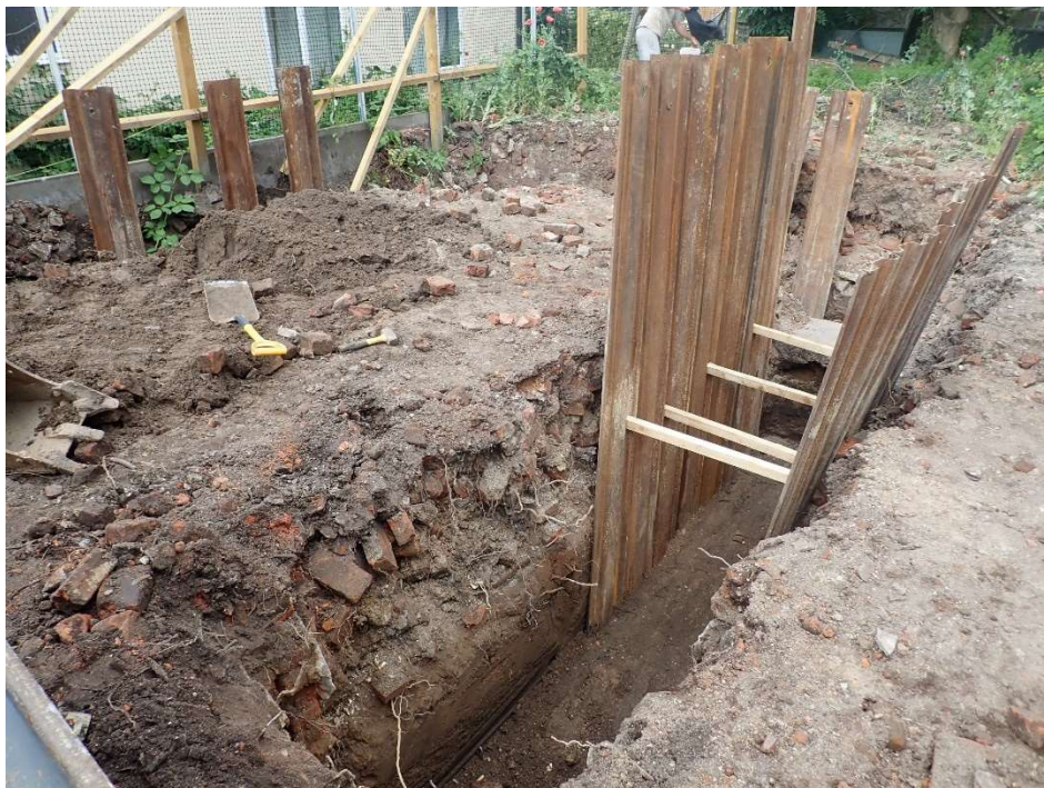
Plate 7. Placing sheet piling in the footings, looking north
