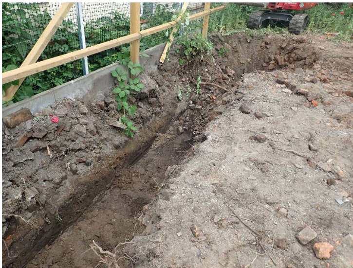
Plate 2. The west side footings, looking north
