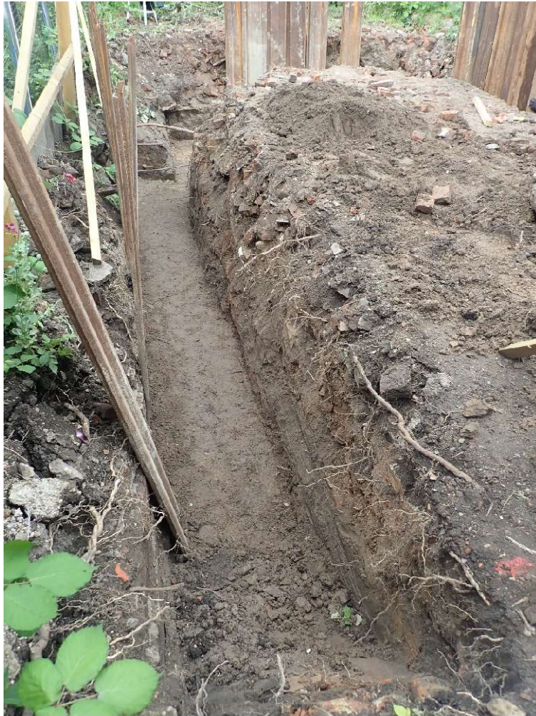
Plate 6. The west side footing, looking north
