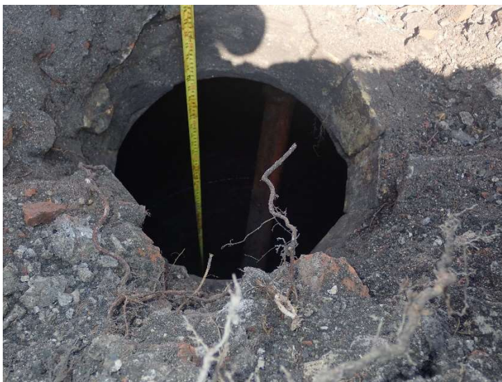
Plate 3. View into cistern 008
