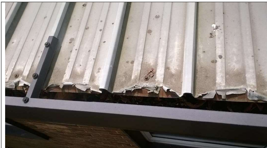
Plate 2: Steel Sheet Roof Covering as Existing (ROOF AREA 1 on plan)
