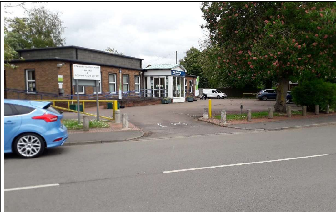
Plate 1: Long Sutton Library viewed from Swapcoat Lane.
