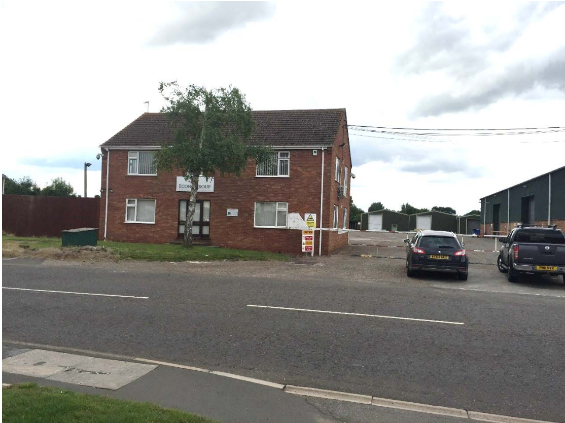
Existing offices and access from Station Road.
