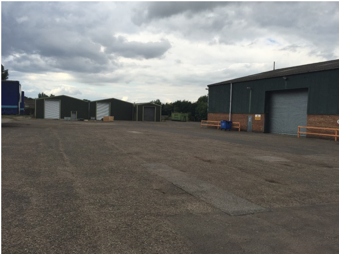
Looking north within the site at the existing industrial buildings.
