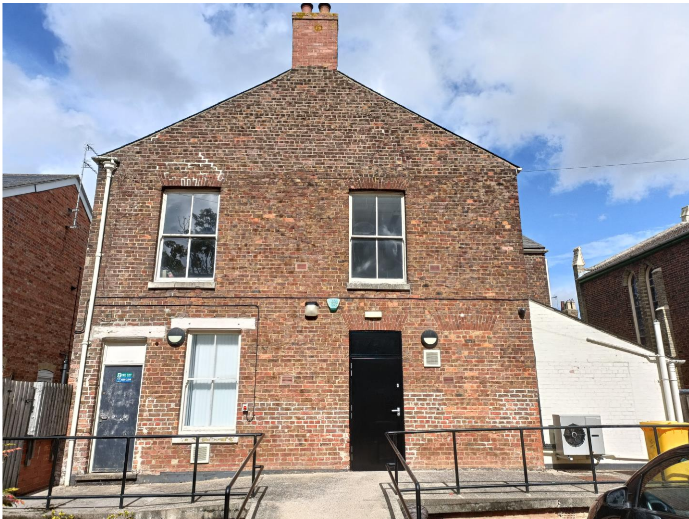
View 1 looking north toward the rear of the building, from the rear car park area.
