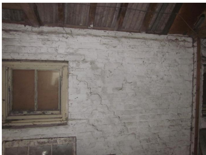
Photograph # 17 (Rear Elevation – First Floor)
