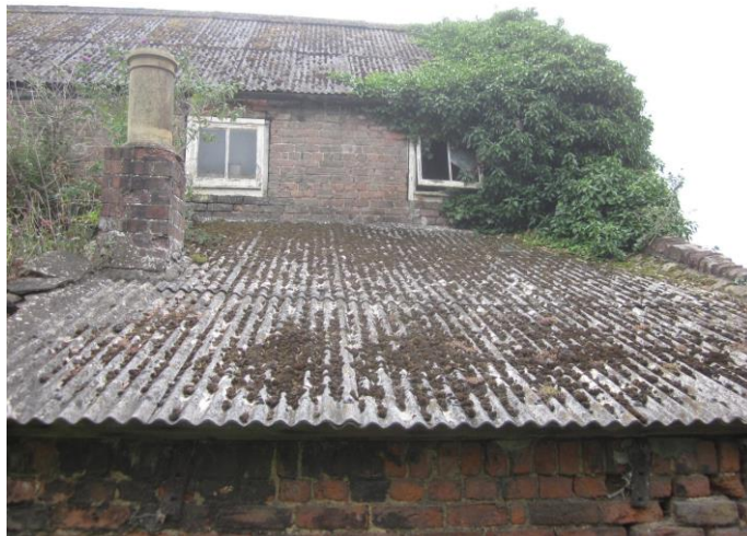
Photograph # 5 (Part Rear Elevation / Single Storey Roof)
