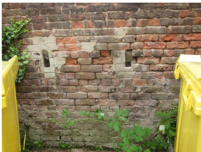
Photograph # 12 (Pockets in Gable Wall)
