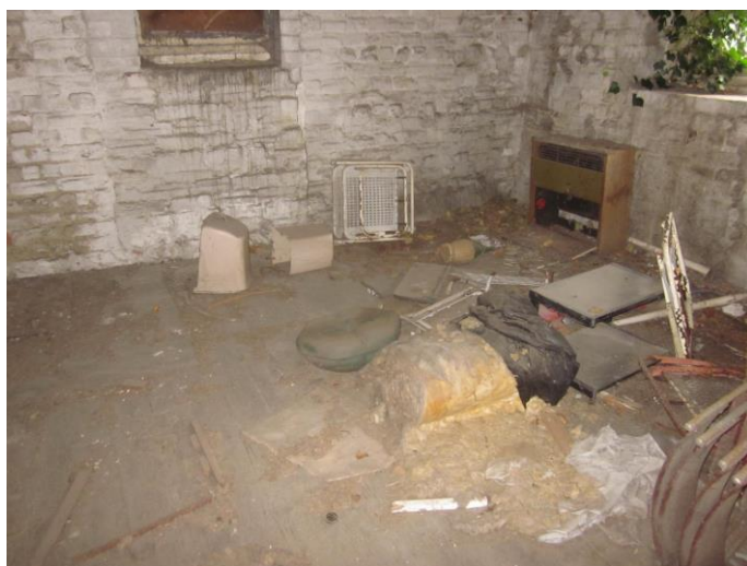
Photograph # 18 (Rear / Gable Elevation and First Floor)
