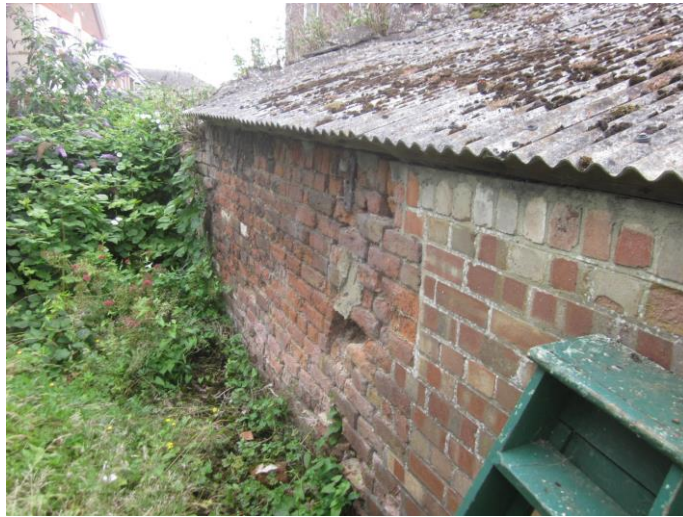
Photograph # 7 (Single Storey Rear Projection)
