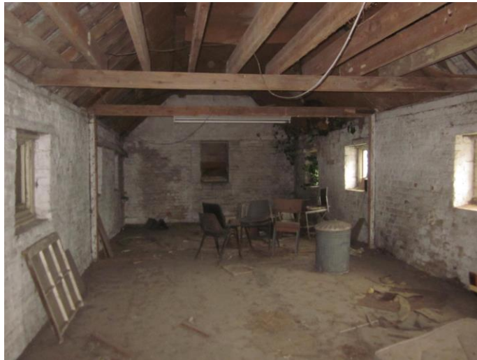
Photograph # 13 (First Floor / Roof)
