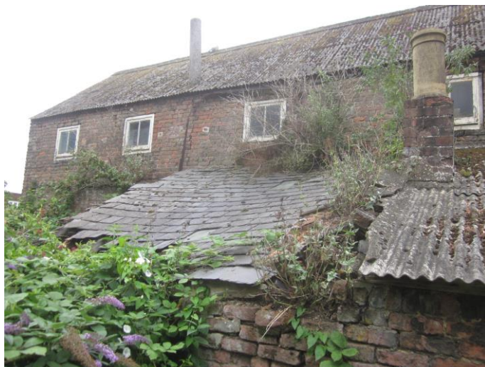
Photograph # 8 (Single Storey Rear Projection)
