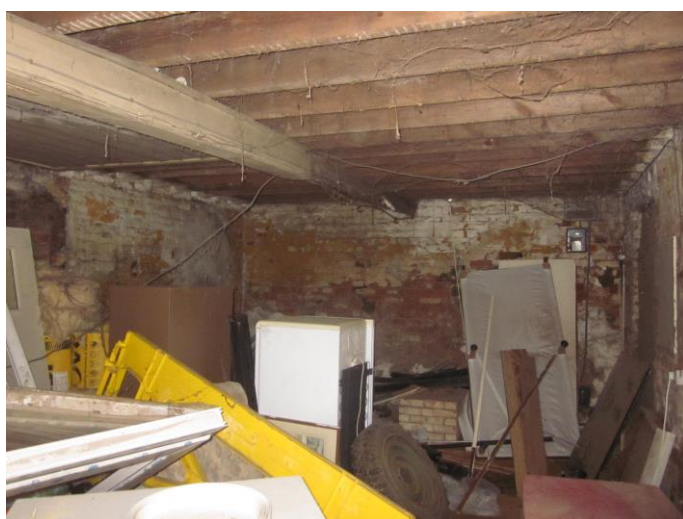
Photograph # 20 (Underside of First Floor – Overspanned Beams)
