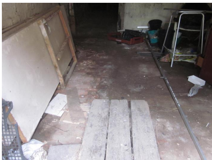
Photograph # 23 (Typical Ground Floor / Tiles)
