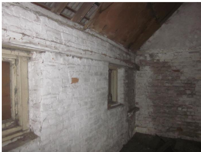
Photograph # 15 (Roof / Eaves)
