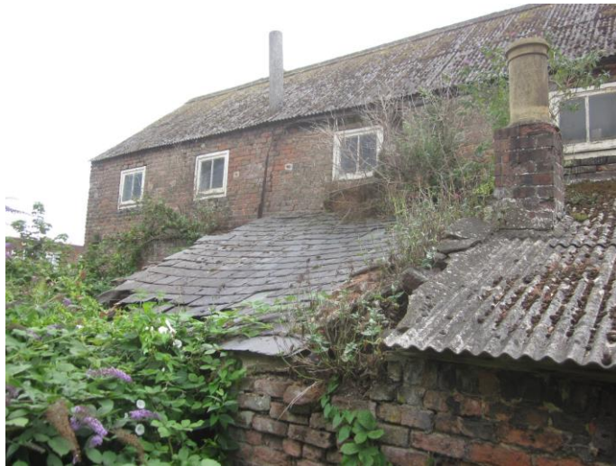
Photograph # 4 (Part Rear Elevation / Single Storey Roof)
