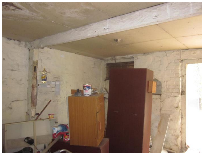
Photograph # 22 (Ground Floor / First Floor Support Beams)
