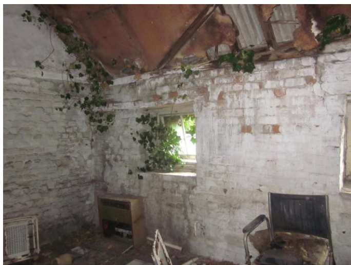
Photograph # 16 (Rear Elevation – First Floor)
