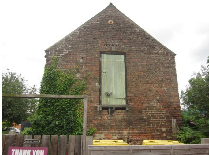
Photograph # 3 (Gable Elevation – Facing Residential Home)
