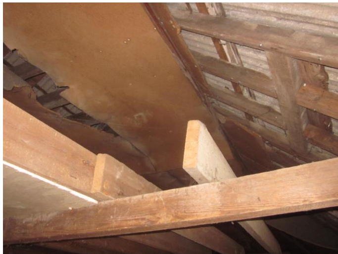
Photograph # 14 (Typical Roof)
