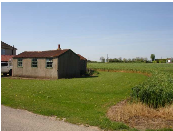
View of site from Gimmels Gate
