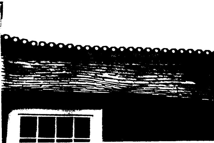
5. NORTH ELEVATION ROOF SLOPE
