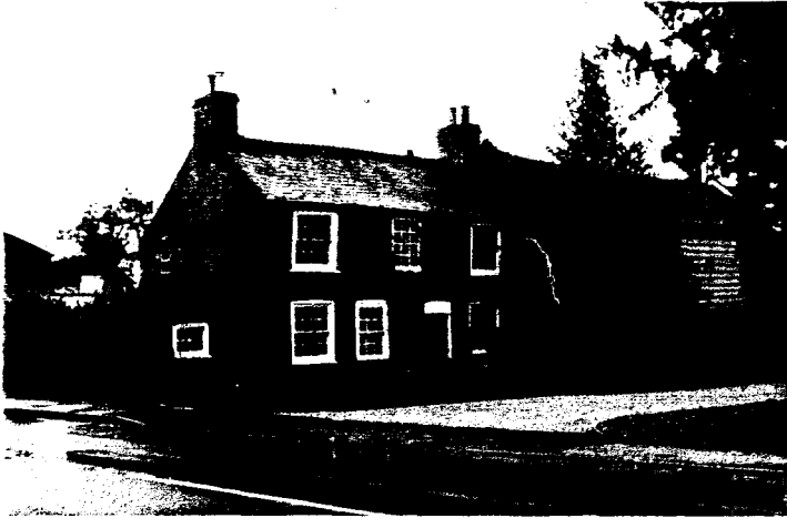
1. NORTH ELEVATION- GENERAL VIEW
