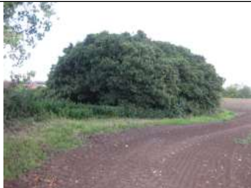
8 – Ivy-covered building B1
