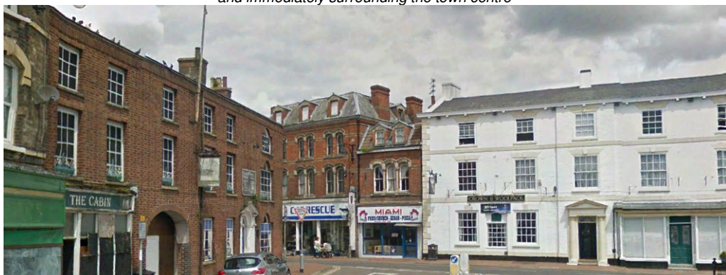
Photos below and on following page showing some of the 3.5 storey buildings within, and immediately surrounding the town centre
