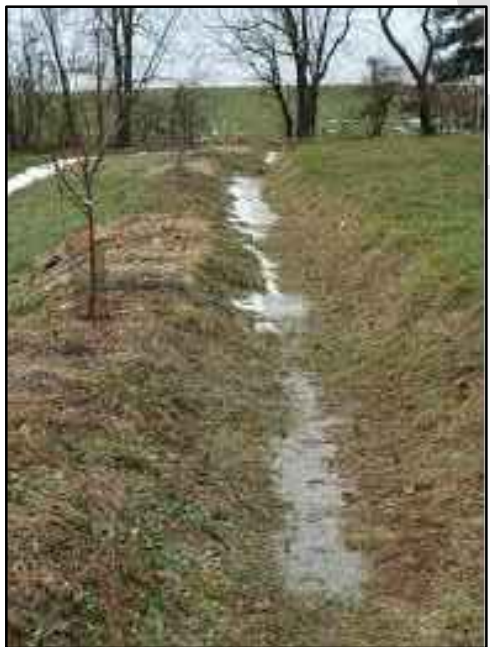
EXISTING DITCHES UTILISED FOR SWALE / WATER RETENTION
