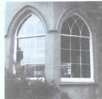
Grade II Listed Building - Gothic Style Windows
