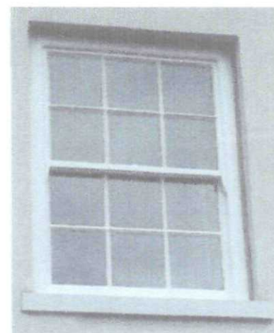
Grade II Listed Building - Surrey
