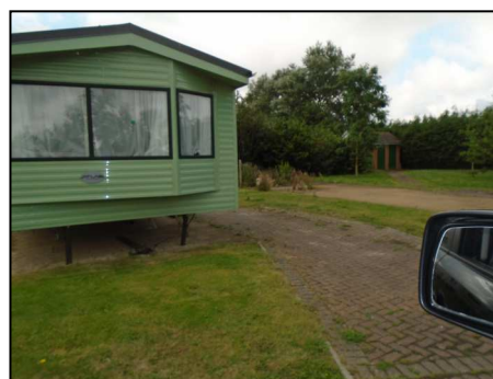
Photo 7 Possible Pump House (1) (Area A)
