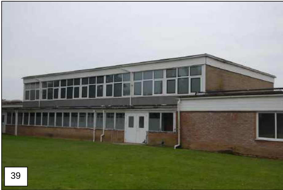
Library The corridor along the south side of the Library is of mixed pink & red bricks, with a series of single fixed lights with timber window frames, (brick size:, 215mm x 100mm x 65mm; 3C = 9") in stretcher bond. The western extension of this corridor with its wide UPVC fascia is in red rusticated brick. The Library windows are UPVC replacements, and the rectilinear framing of the original design has been lost.
