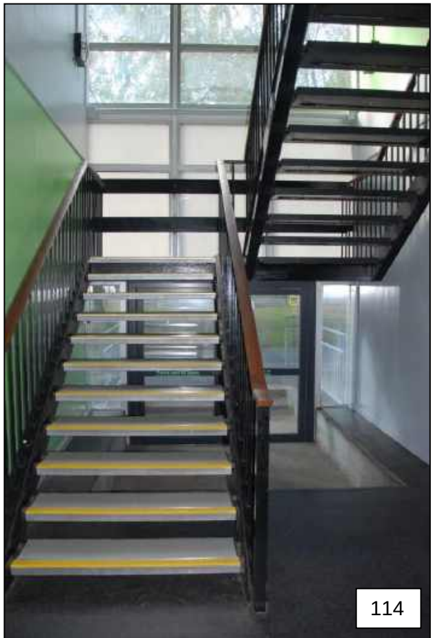
West Stairwell The staircase at the west side is of identical materials and construction as that described to the east.
