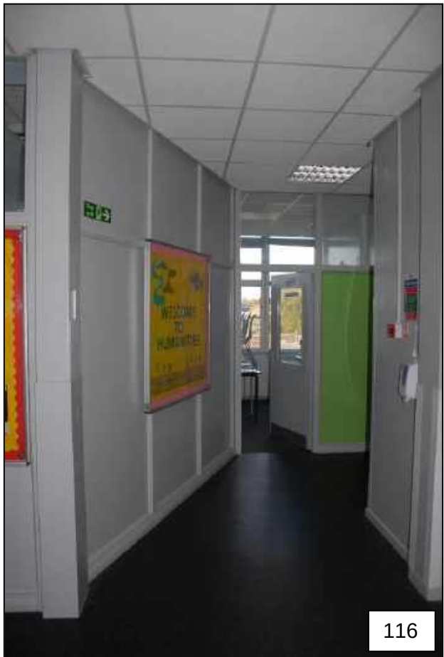
1F Corridor The first-floor corridor deflects north to the landing of the eastern staircase, resulting in the eastern classroom having a diagonal SW corner.
