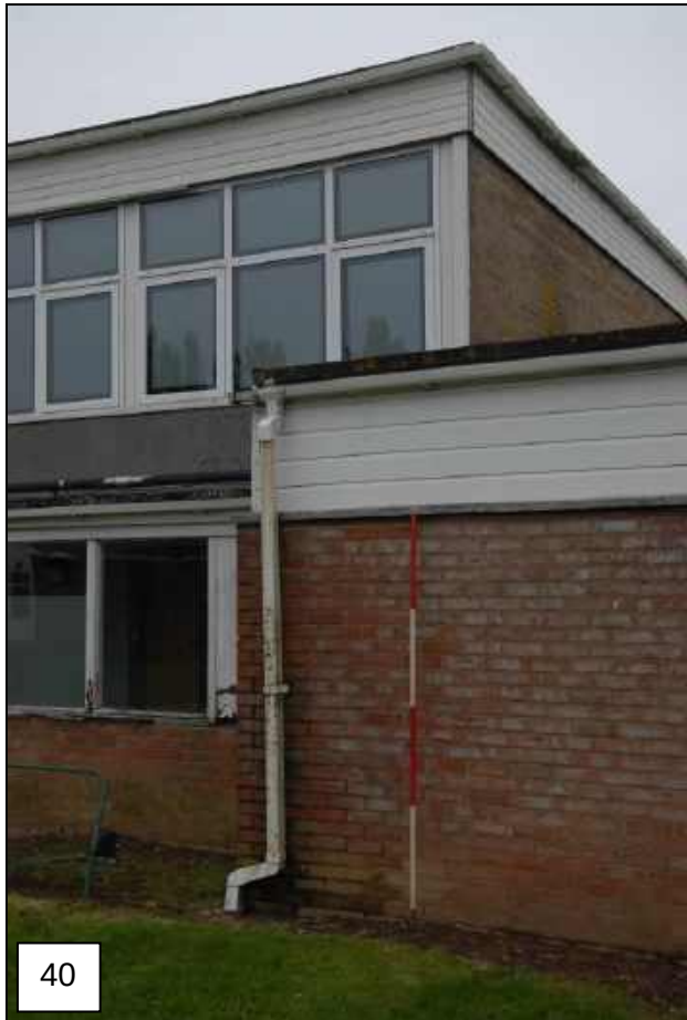
Library The corridor along the south side of the Library is of mixed pink & red bricks, with a series of single fixed lights with timber window frames, (brick size:, 215mm x 100mm x 65mm; 3C = 9") in stretcher bond. The western extension of this corridor with its wide UPVC fascia is in red rusticated brick. The Library windows are UPVC replacements, and the rectilinear framing of the original design has been lost.
