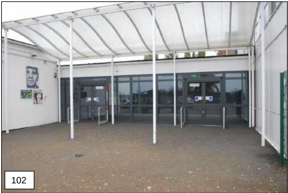
A single-storey linking block at the east side houses the main entrance to the school: this has a modern UPVC glazed partition similar to the glazing of the Dining Hall with a UPVC and steel external canopy.
