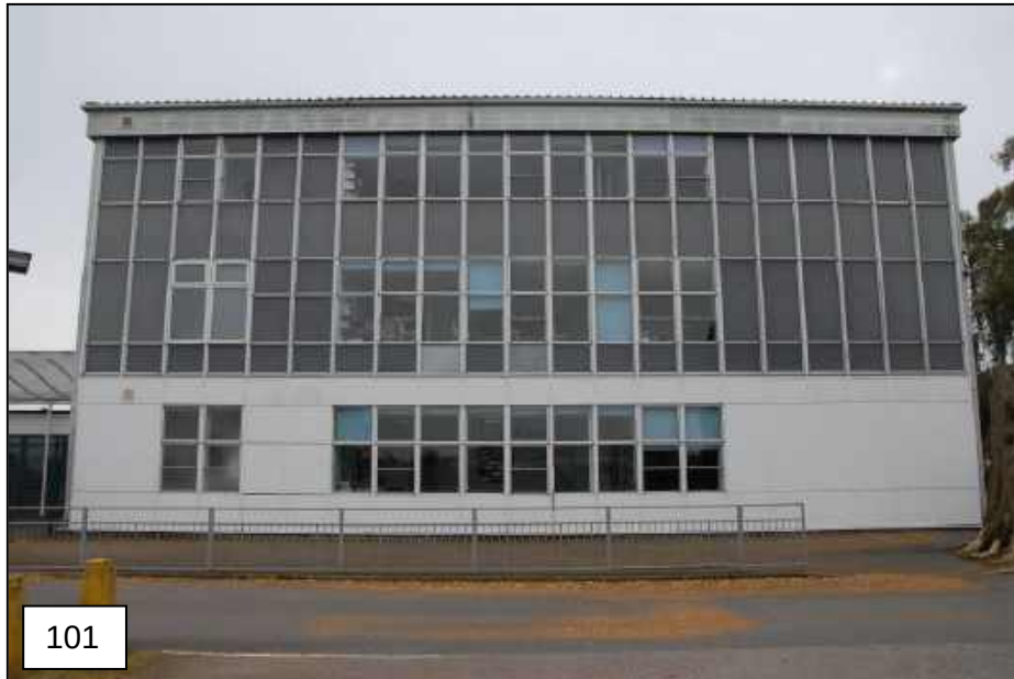
North Side This has a blind western bay and some UPVC replacement windows; the eastern bay is also partially panelled.
