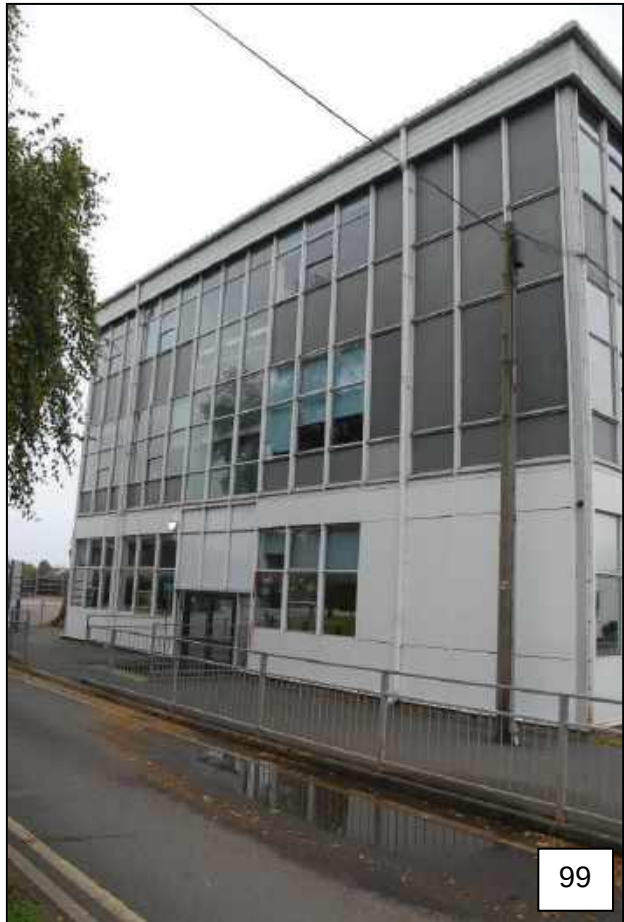
West Side This has a blind southern bay and central ground-floor fire doors..
