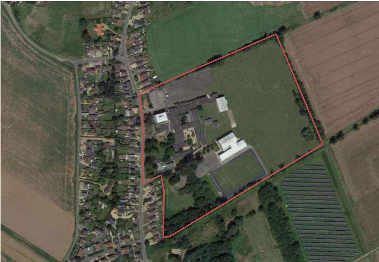
AERIAL IMAGE OF EXISTING SITE LAYOUT
