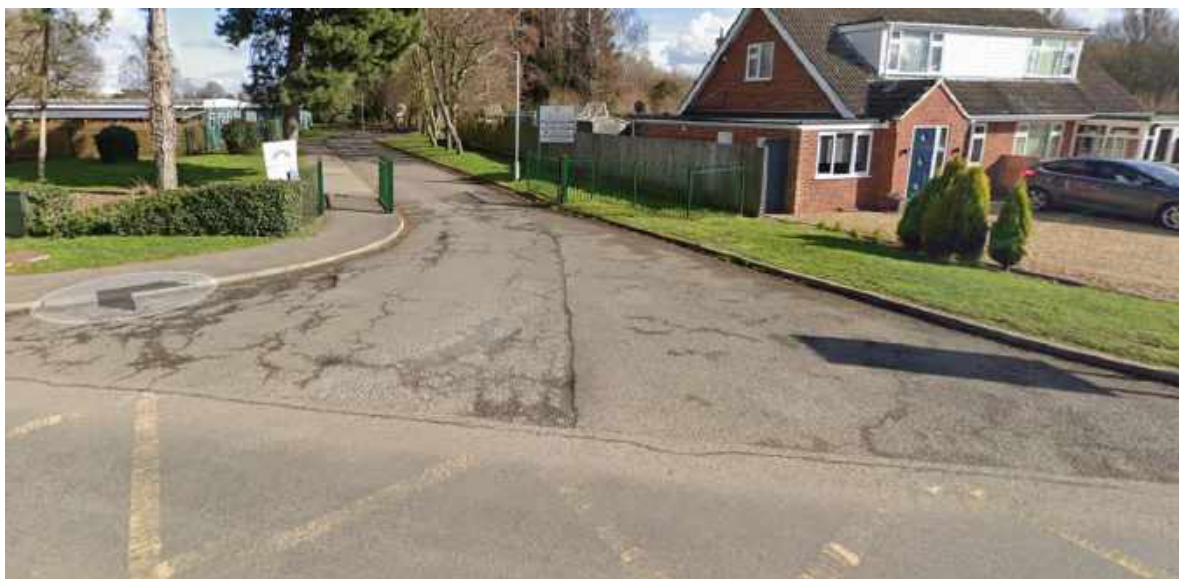
Fig. 3 - Existing Entrance off Little London to Leisure centre
