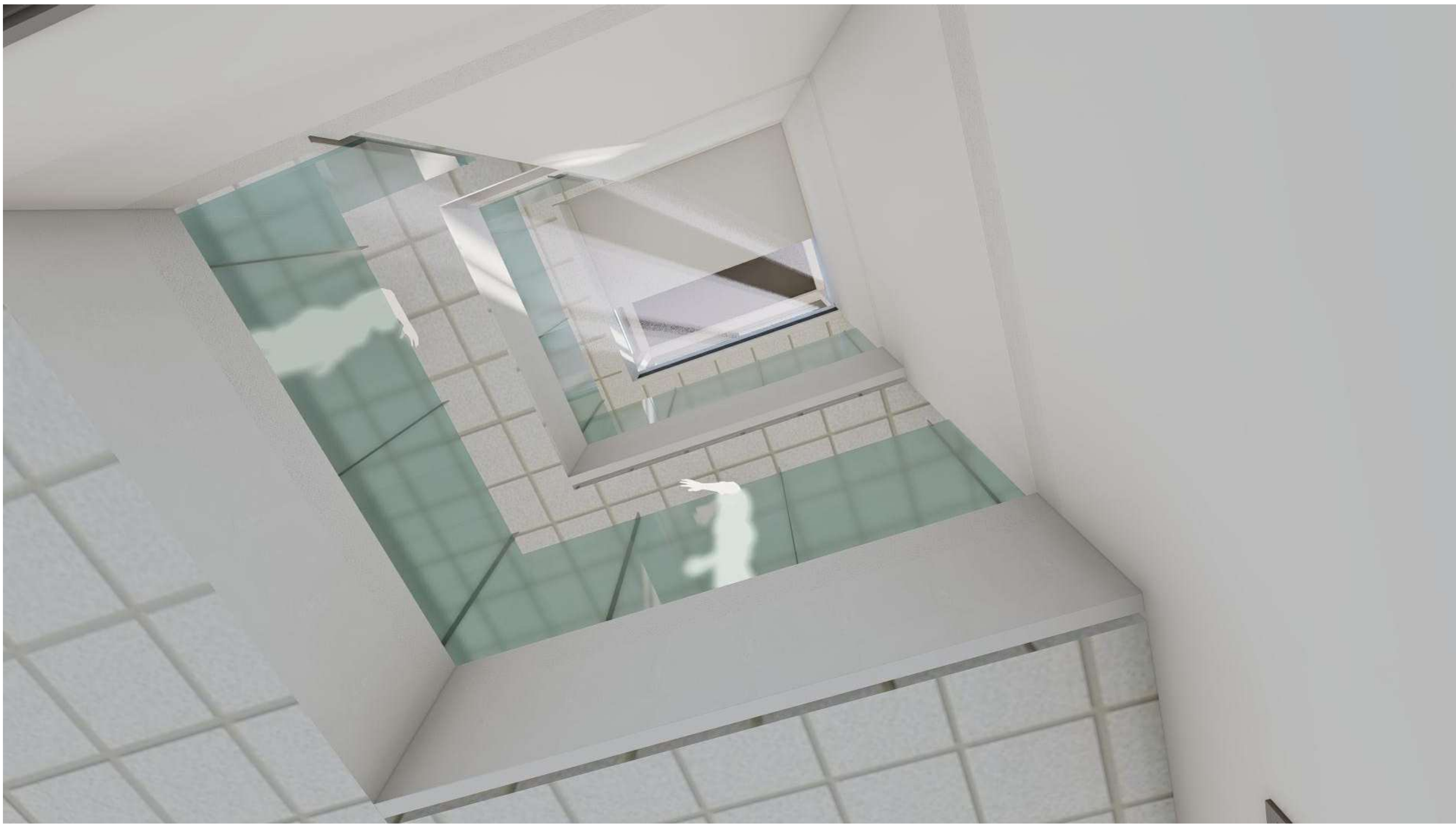
VENTILATION VOID AN TURRET
