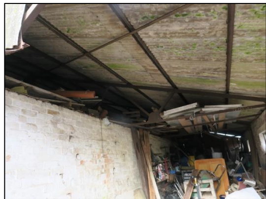
Photograph 6: Representative image showing the rear lean-to structure.
