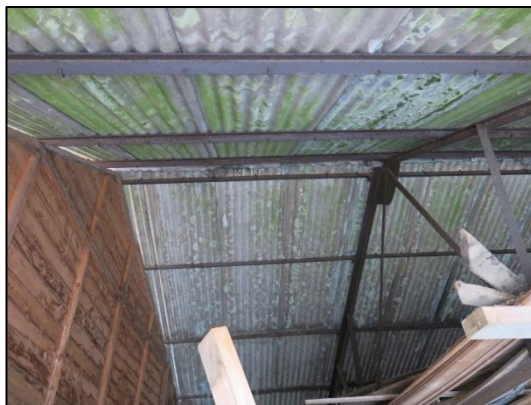
Photograph 5: Representative image showing the metal-framed roof structure.
