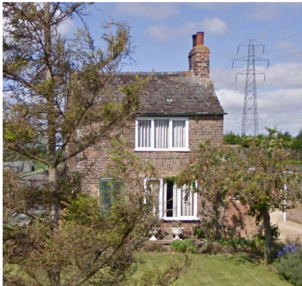
2009 enlargement of Google Maps picture of property highlighting the original arched head to a smaller ground floor window with contrasting brick infill over new window
