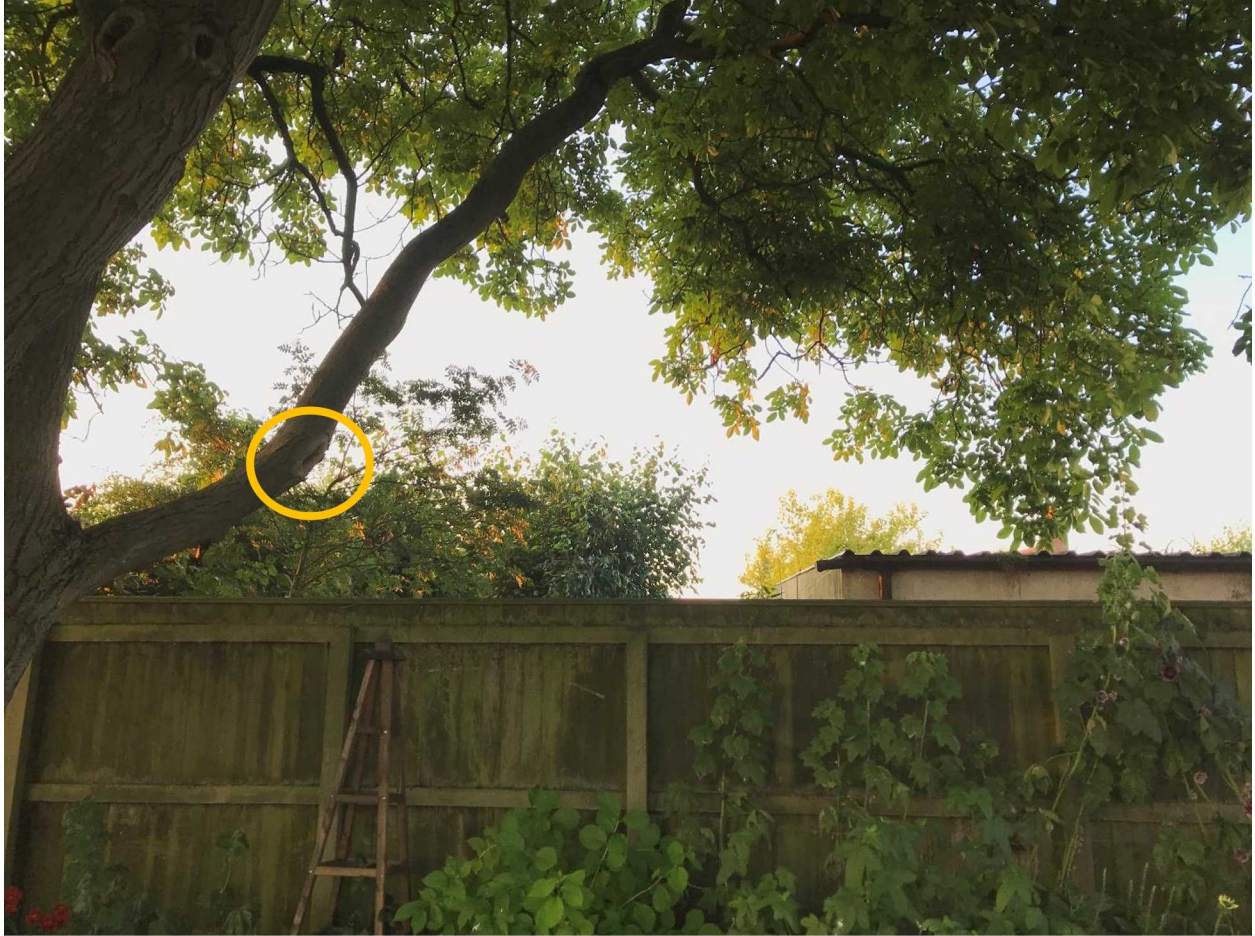
Figure 4: This image highlights the existing wound that is a weak point to this North East overhanging limb that could pose a significant risk if it were to fatigue, potentially causing extensive damage to the neighbour's property.
