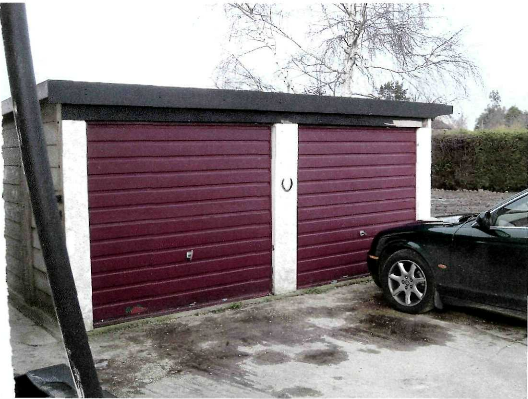
Garage to be demolished
