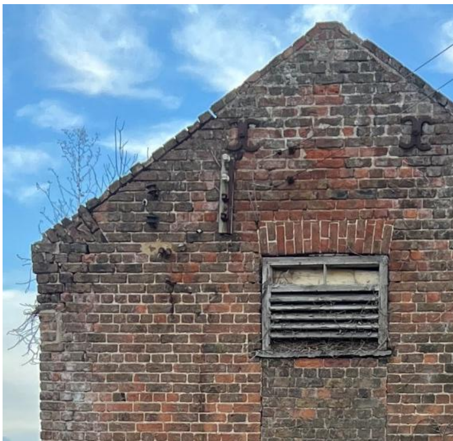
Parapet gable with tumbled brickwork towards eaves, brick on edge detail. Tie rods and infilled opening.
