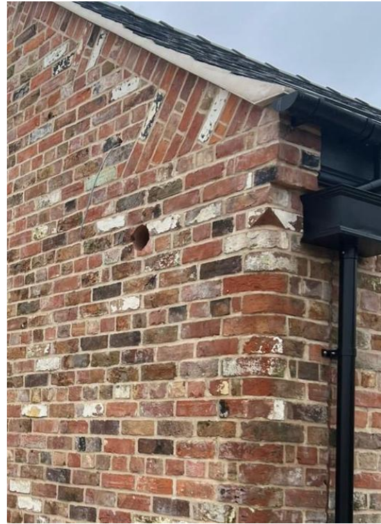
Right: Example of applicants work on another clients project indicating tumbled brickwork and bullnose corner.
