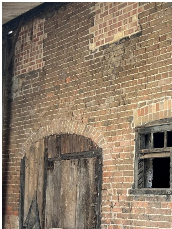
Parabolic arch, double header window heads & infilled openings seen on an internal/enclosed elevation of the existing barn
