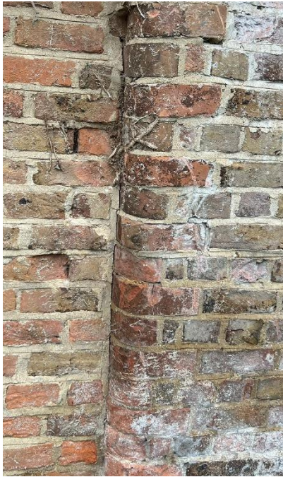
Bullnose corner brickwork to former openings
