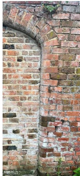
Bullnose corner brickwork to former openings
