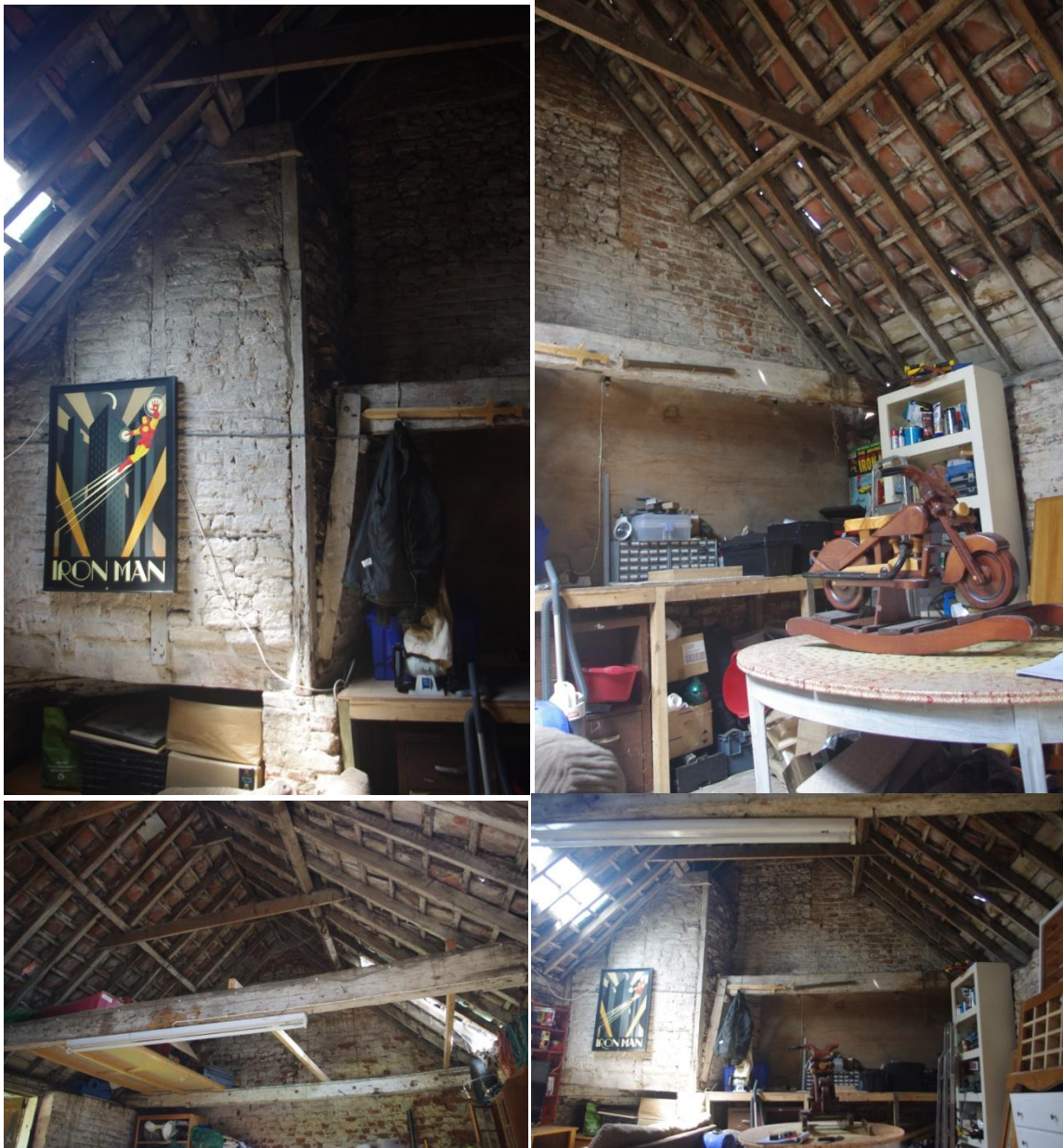
Images from within the outbuilding
