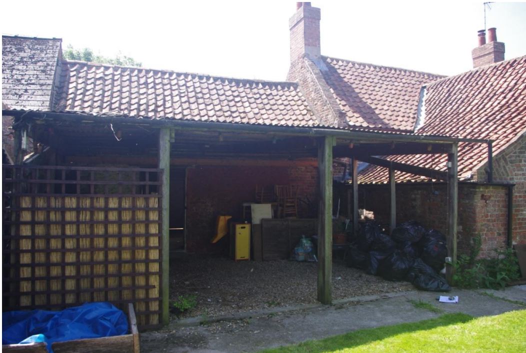
Image above shows the covered timber store to be replaced from the rear garden
