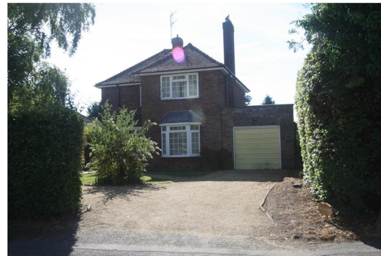
Existing two storey dwelling on Broad Lane
