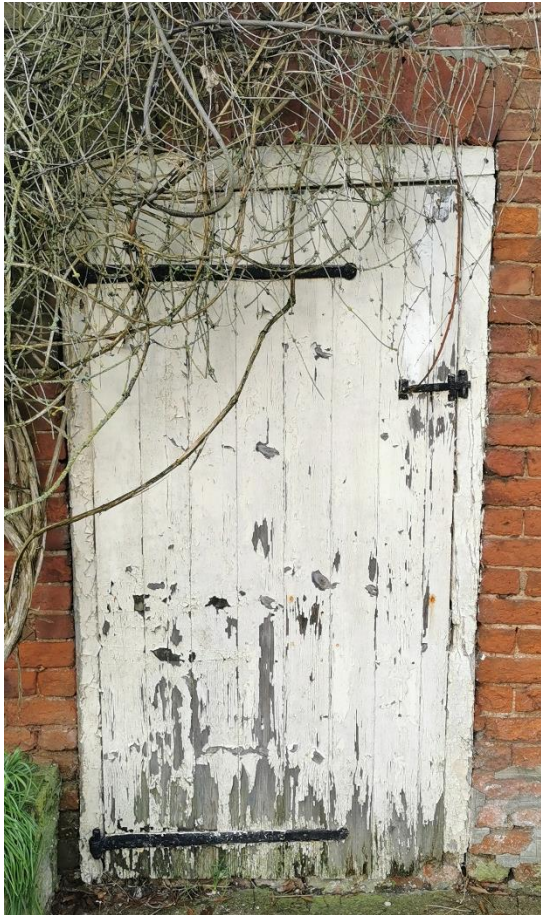
External doors to stables, possibly original although hinges etc have been replaced in places. Left: front elevation with brick arch over, right: side (NE) elevation with timber lintel over
