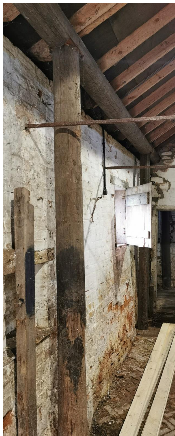
Timber posts installed to support the new modern roof structure seen both externally to the rear and internally to the front
