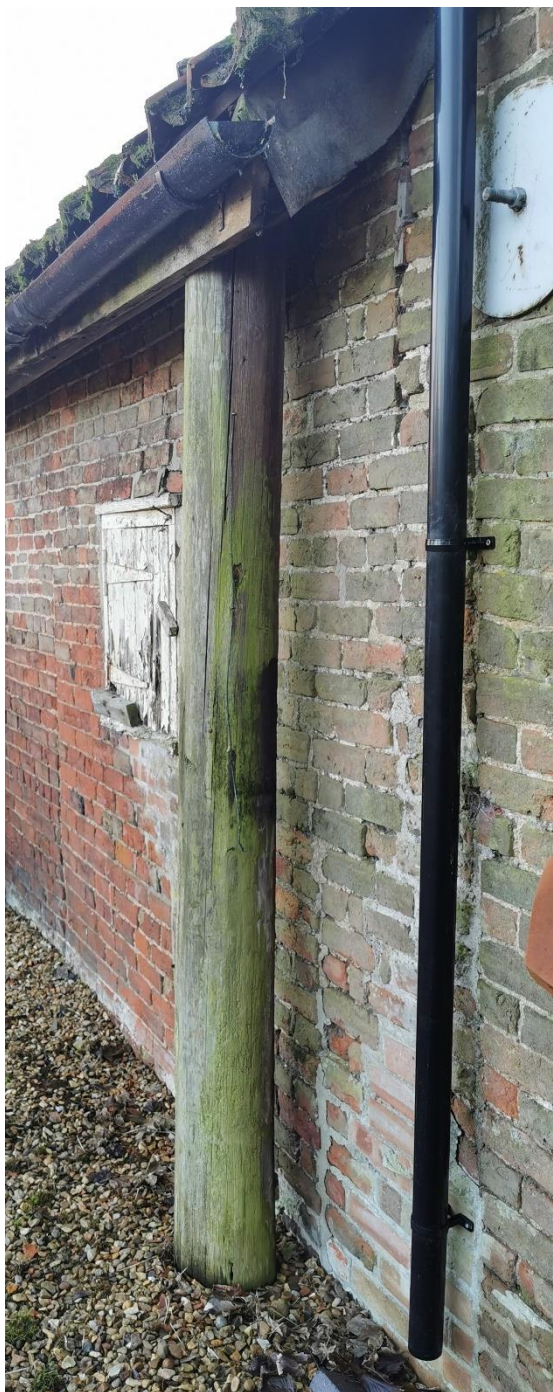
Timber posts installed to support the new modern roof structure seen both externally to the rear and internally to the front
