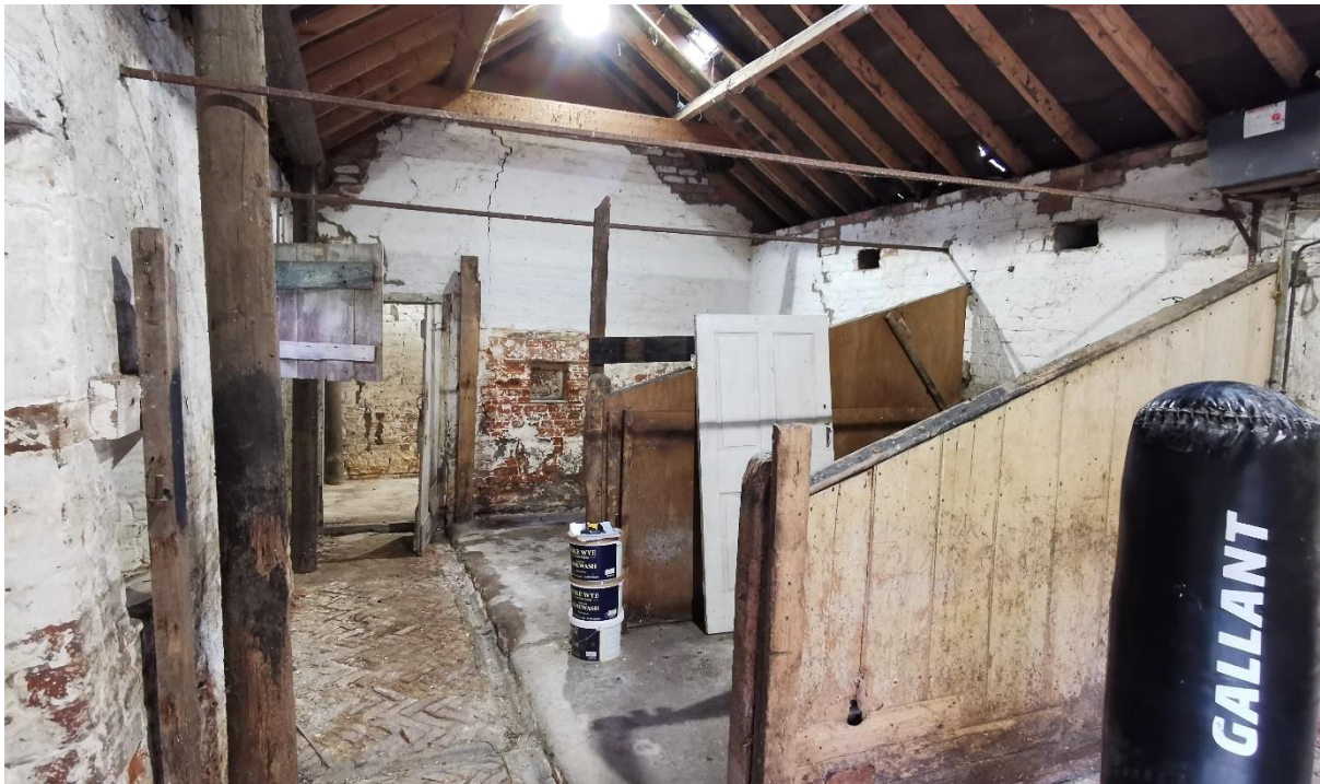
Overall internal view of stable area showing the original floor and stable partitions
