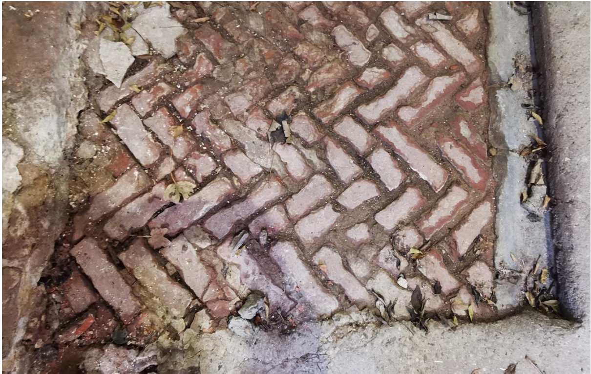
Detailed image of brick herringbone floor
