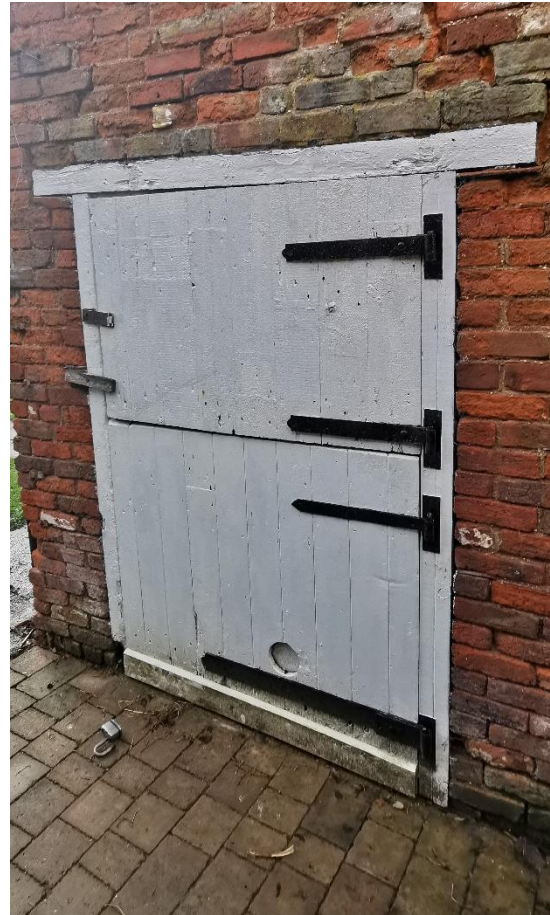
External doors to stables, possibly original although hinges etc have been replaced in places. Left: front elevation with brick arch over, right: side (NE) elevation with timber lintel over
