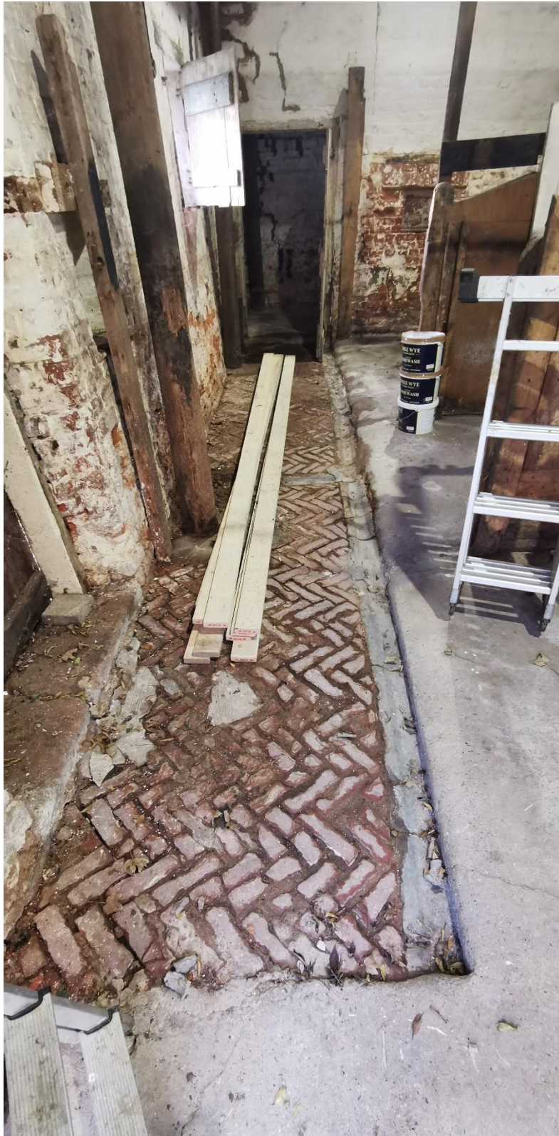
Overview of the original brick herringbone floor with drainage channel to central drain
