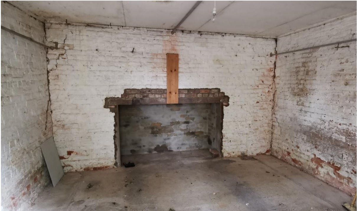
Overall internal view of later added garage, including later step out with timber beam over, as can be seen on the rear elevation
