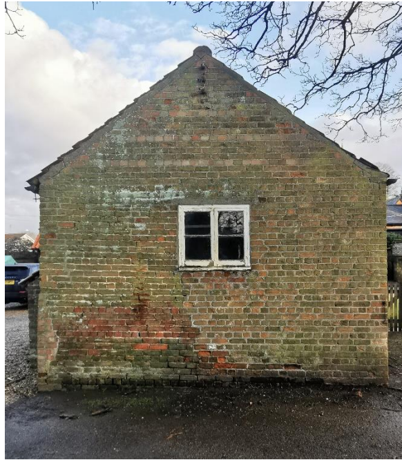
Overall view of side (south west) elevation
