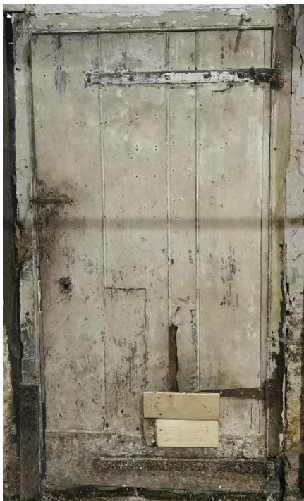
External doors to stables, possibly original although hinges etc have been replaced in places. Left: front elevation with brick arch over, right: side (NE) elevation with timber lintel over
