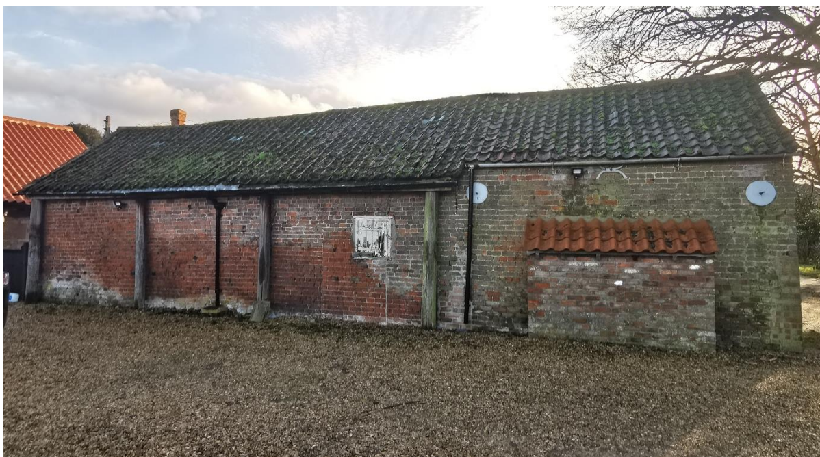
Overall view of rear (north west) elevation showing the small addition to the rear of the garage and the timber posts supporting the modern roof structure
