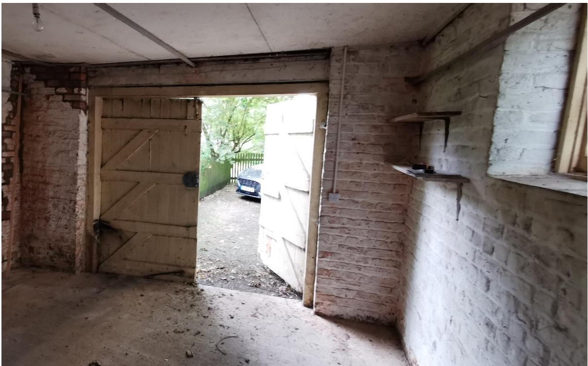
Internal view of garage showing doors to front elevation and window to side (SW) elevation
