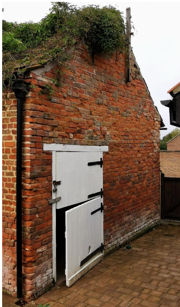
Overall view of side (north east) elevation
