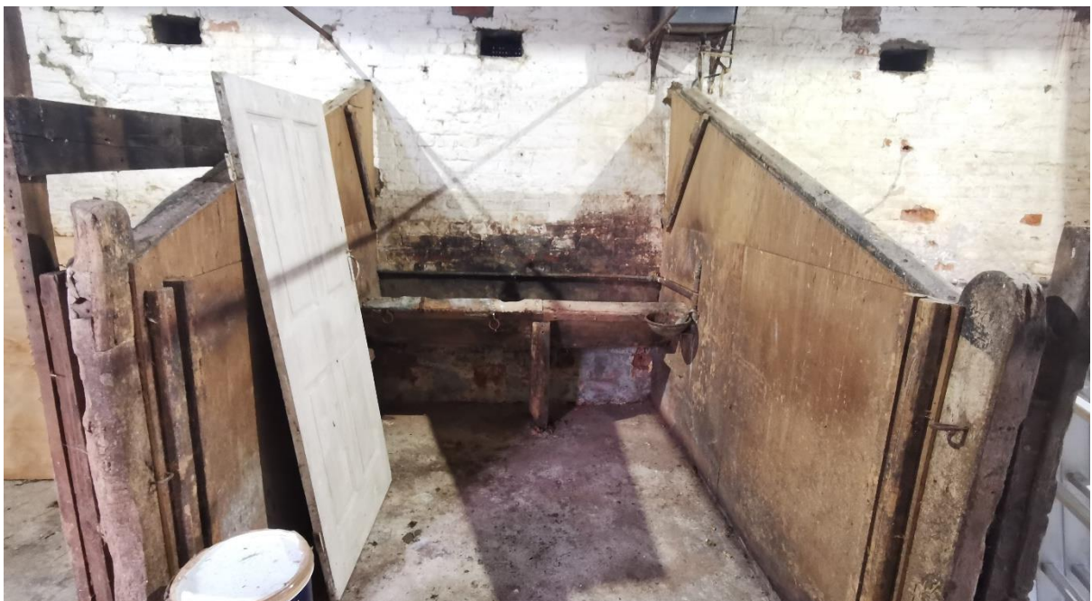
View showing central stable with existing timber partitions and feeding trough
