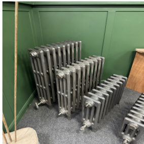
New Raditors To Replace the modern 20th Century Style. All Rooms except those areas with underfloor heating
