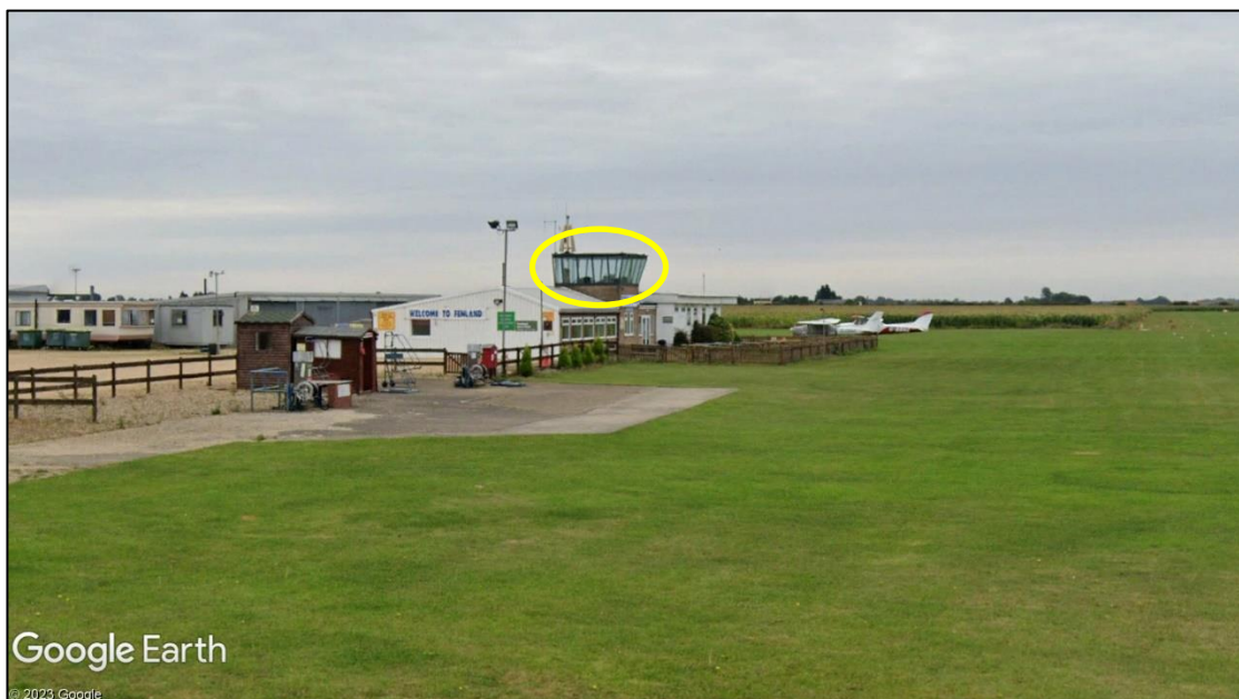
Figure 24 Ground-based view of the ATC Tower (the visual control room is circled)
