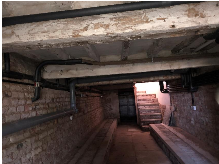
Figure 3-1 Inside the Basement
