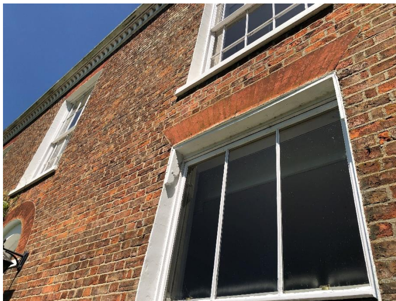
Figure 4-1 External Window Header
