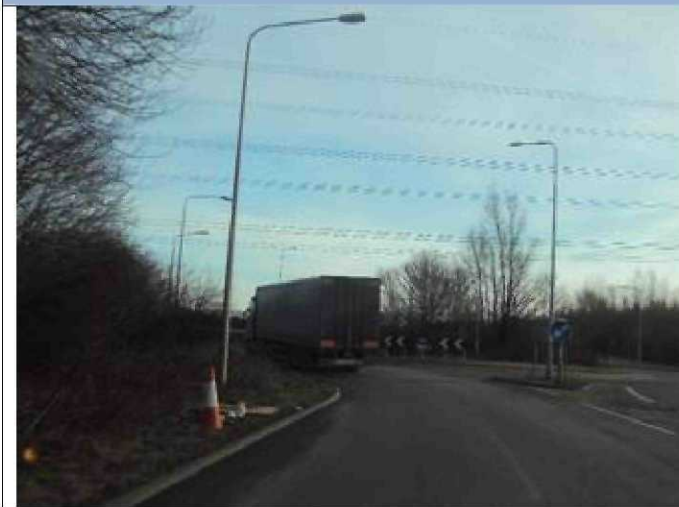
7.4.2.1. – Entrance to roundabout
