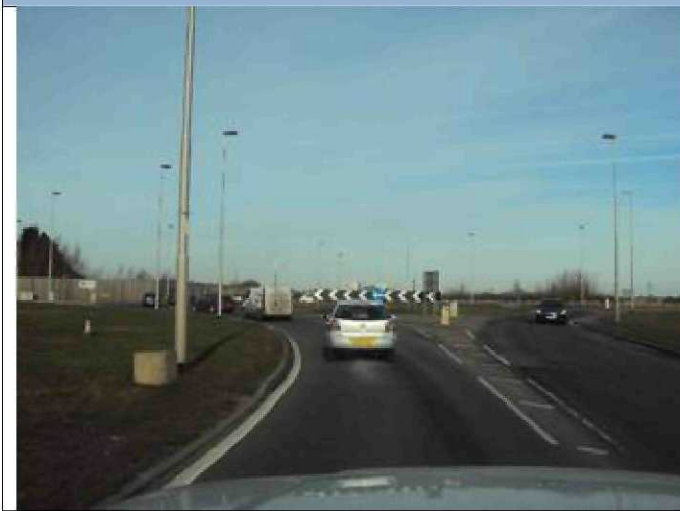
7.7.1.1. – Entrance to roundabout
