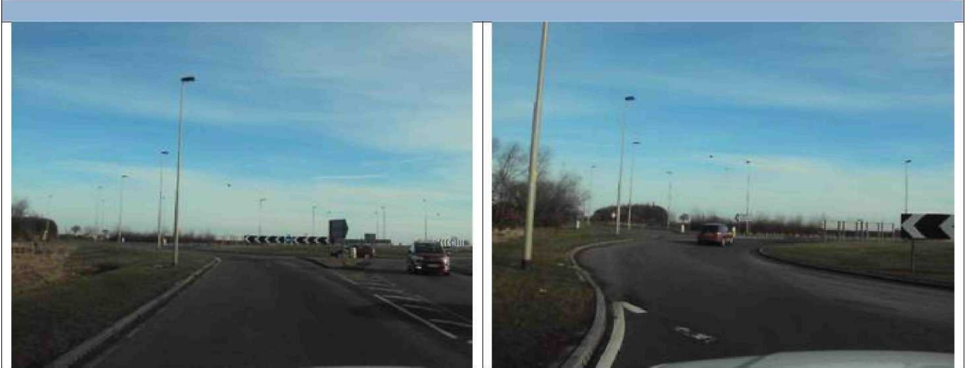
7.6.1.1. – Entrance to roundabout
