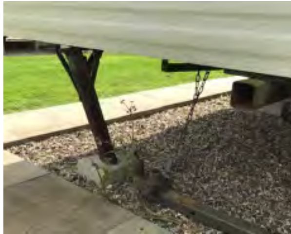
Typical Anchor Chains
