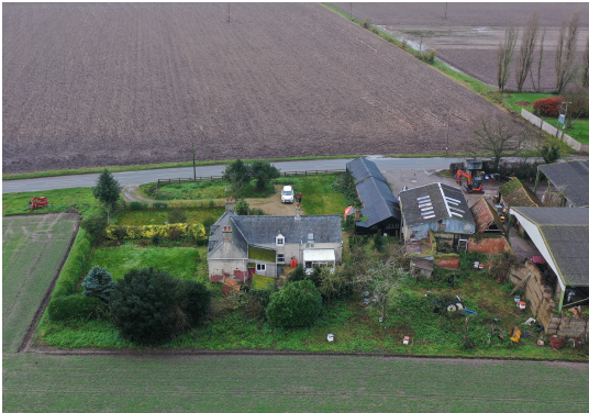
Fig 05. Aerial view from east.
