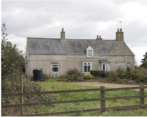
Fig 03. West elevation from Fen Gate
