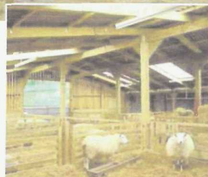
The internal pillars of this supported apex building are ideal for the attachment of internal feed barriers and penning.
