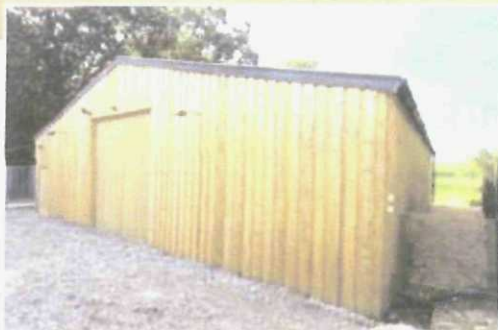
13.790m wide trussed type clear span used as a dog training facility with additional translucent panels in the roof to increase natural light input.
