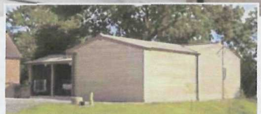
An L shaped trussed type clear span, forming a courtyard effect in conjunction with existing buildings.
