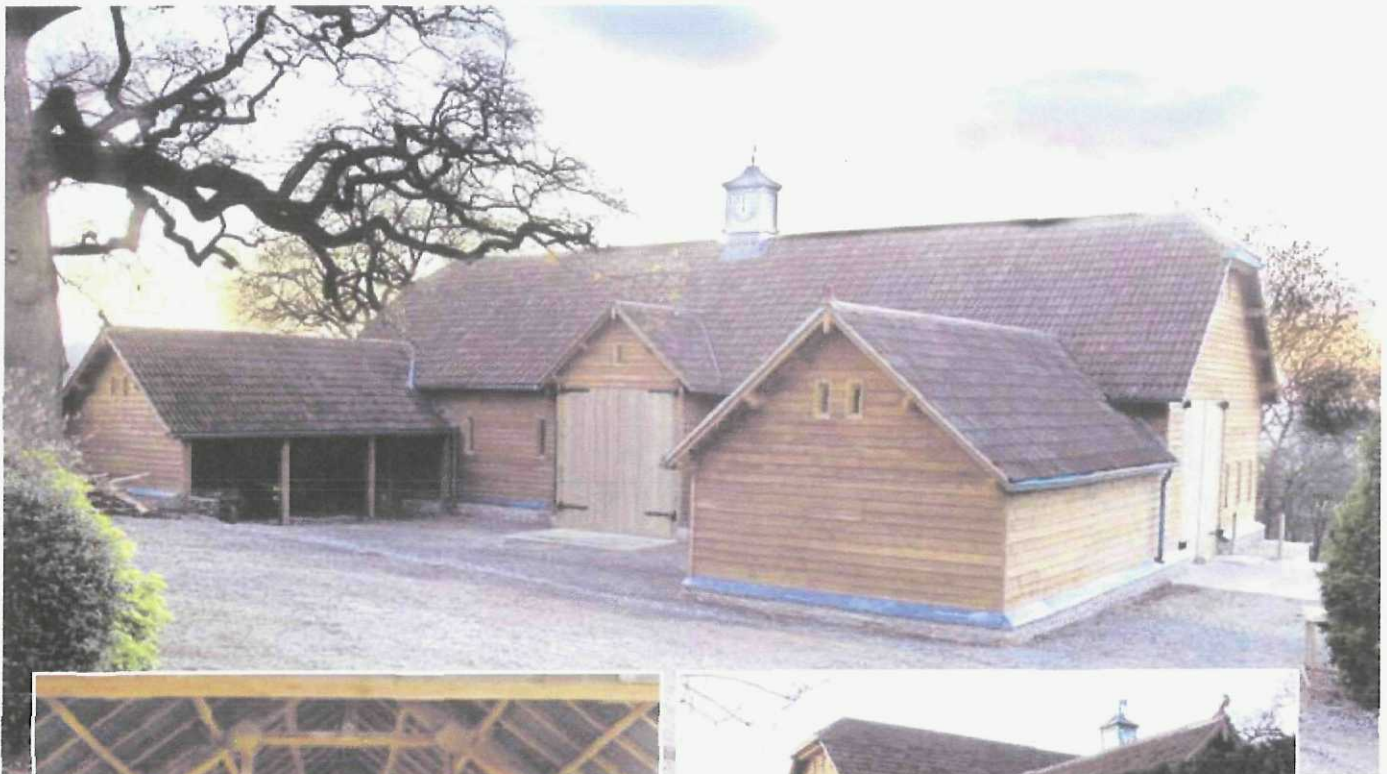
Although adjacent to the house, the use of profiled sheeting on the roof and half gables, provides this building with a barn like appearance to great effect.
