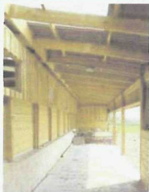
A combination of mono-pitch and supported apex allows for easy access to stables, hay storage and garaging of a horse box.
