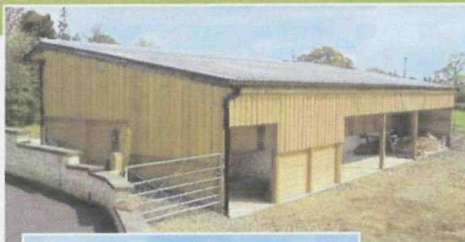
A mono-pitch and supported apex building combined, which provides flexible storage and access to three sides.
