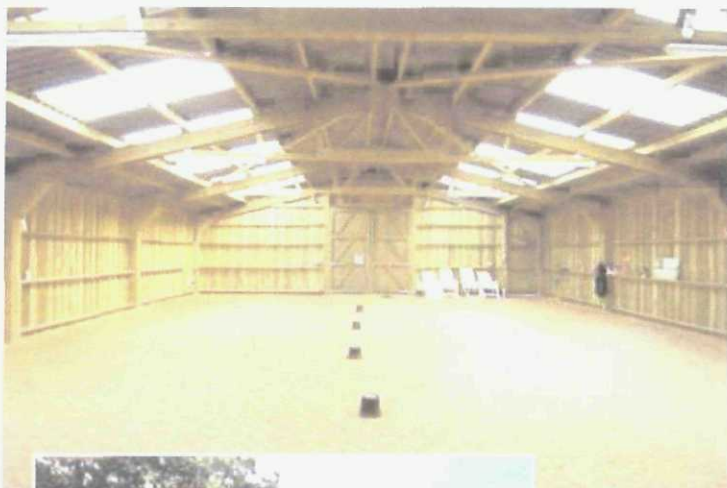
13.790m wide trussed type clear span used as a dog training facility with additional translucent panels in the roof to increase natural light input.
