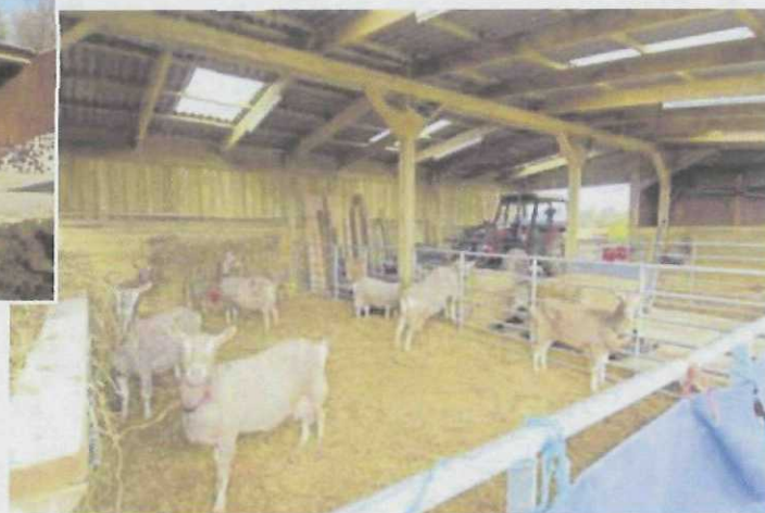
The central pillars on this 9.440m wide supported apex are as robust as the main building pillars, providing support for internal gates and penning.
