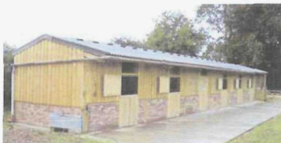
This customer purchased a Farmplus kit building and erected these stables himself.
