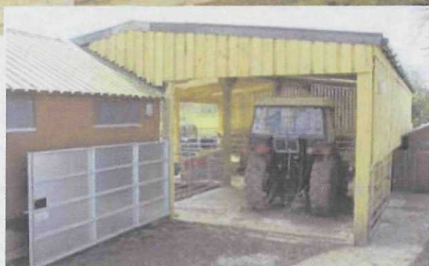
The central pillars on this 9.440m wide supported apex are as robust as the main building pillars, providing support for internal gates and penning.
