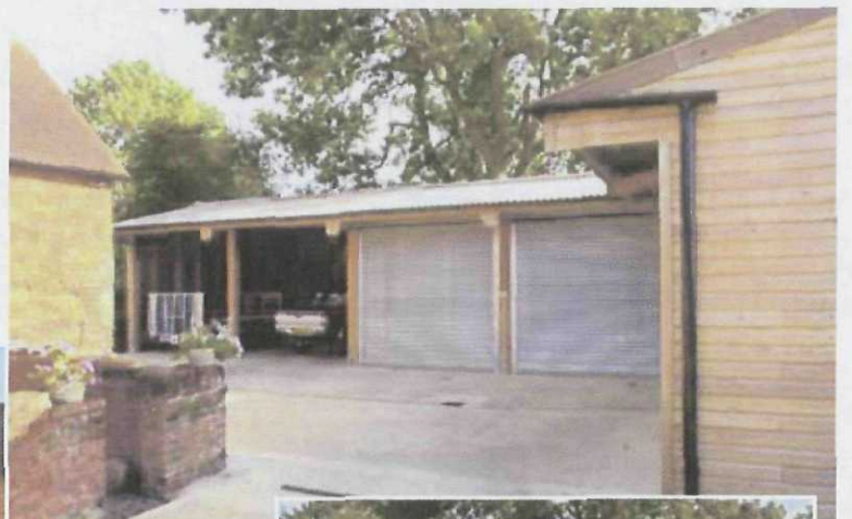
An L shaped trussed type clear span, forming a courtyard effect in conjunction with existing buildings.
