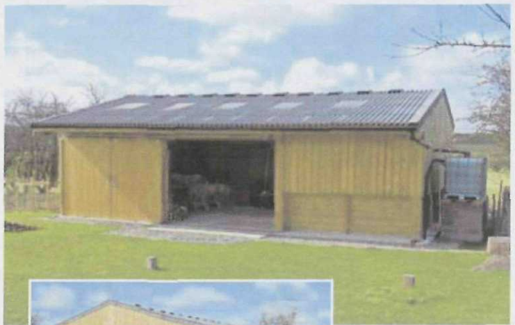
A fully enclosed 6.4m wide trussed type clear span, supplied with a roof cantilever for additional protection on what is an exposed site.
