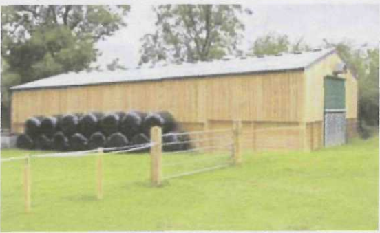
9.150m wide trussed type clear span used to great effect on a small holding, for livestock and general storage.
