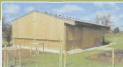
A fully enclosed 6.4m wide trussed type clear span, supplied with a roof cantilever for additional protection on what is an exposed site.
