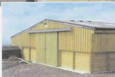
A mono-pitch and supported apex building combined, which provides flexible storage and access to three sides.
