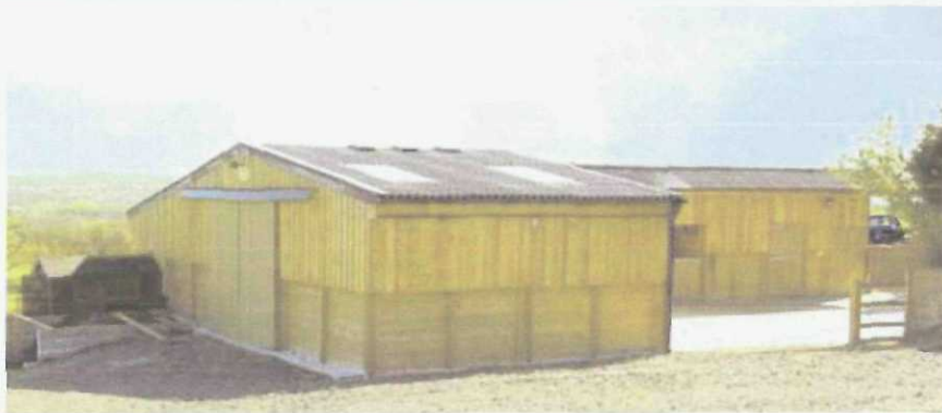
A combination of mono-pitch and supported apex allows for easy access to stables, hay storage and garaging of a horse box.
