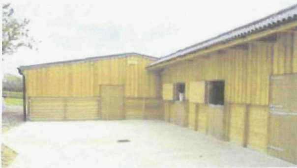
A combination of mono-pitch and supported apex allows for easy access to stables, hay storage and garaging of a horse box.
