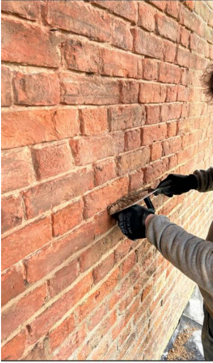
Preparing new pointing ready for bag finish
