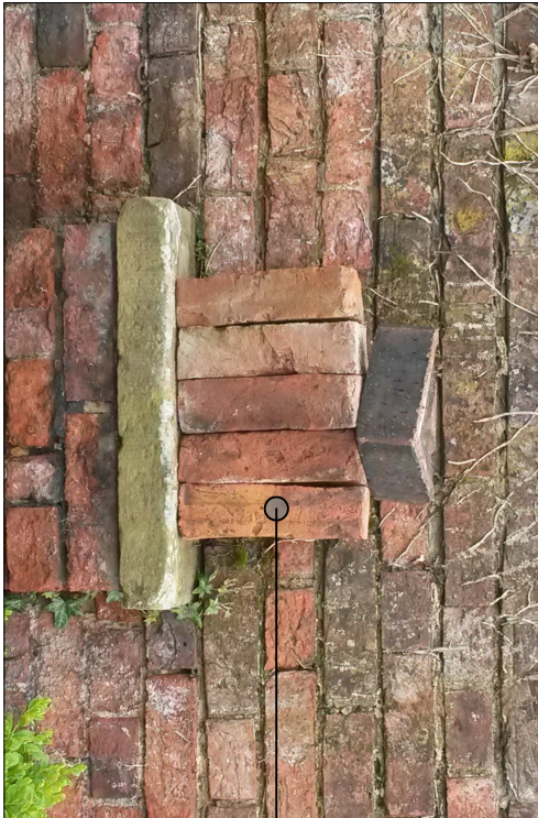
South Lincolnshire Reclaimed Brick from a Building in Tydd St Giles
