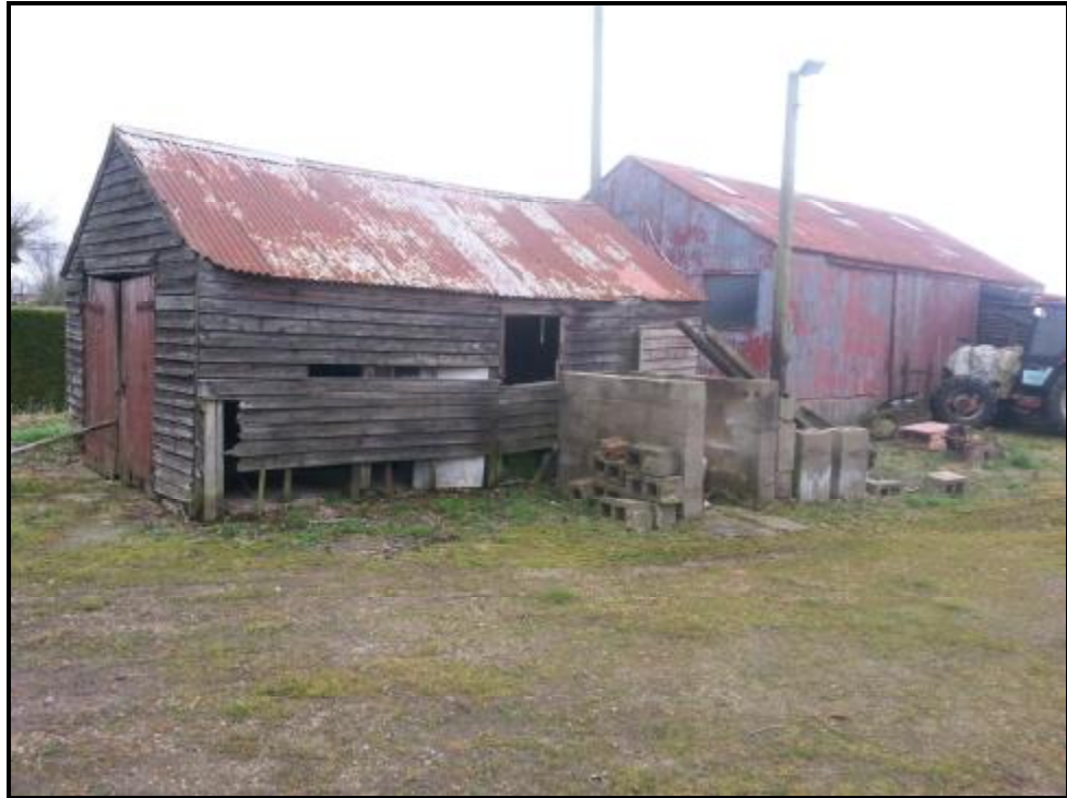
Timber building and potential location of above ground fuel tank
