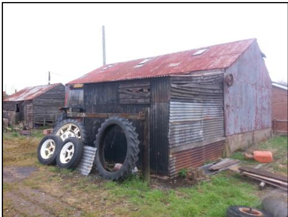
Metal sheeted building
