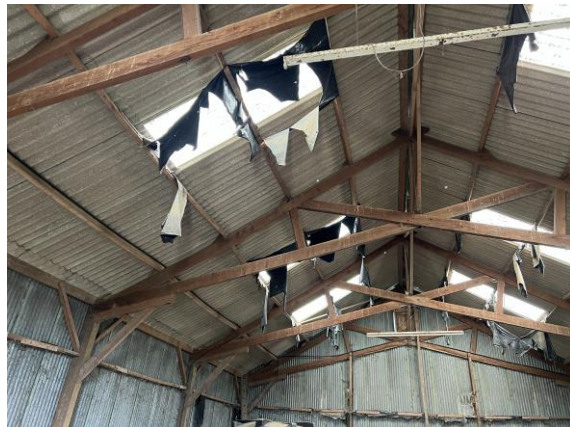
Fig. 2 Agricultural building interior showing timber structure.
