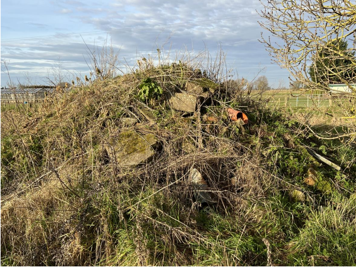
Ph. 3 Detailed view of the pile of building rubble at the north end of the site.
