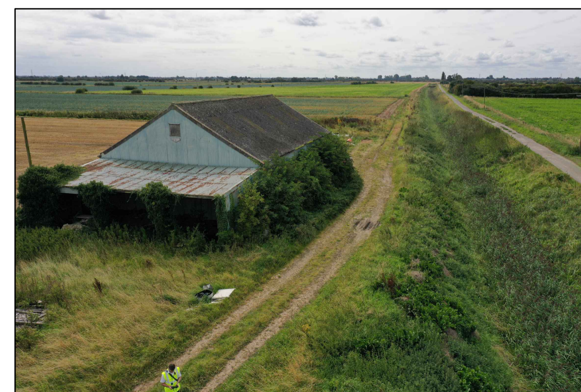
High level view from north west
