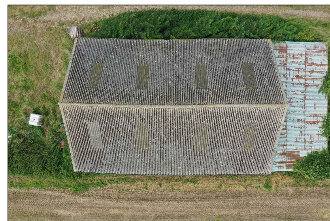
Aerial view of roof
