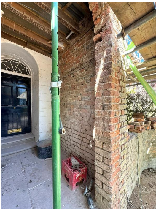
Final Cleaning of bricks and Raking Out of Old mortar
