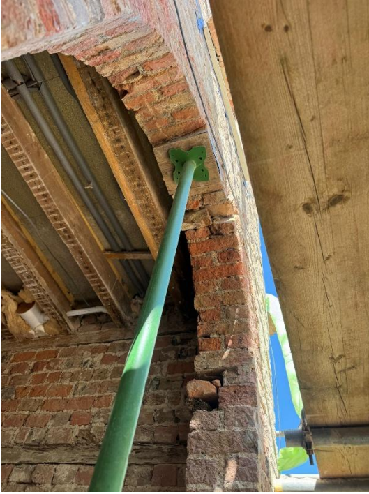
Suspended plasterboard ceiling removed.
