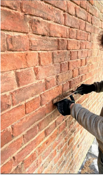
Preparing new pointing ready for bag finish
