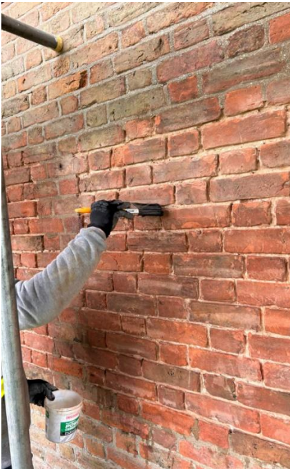
Brushing out loose debris before damping of joints
