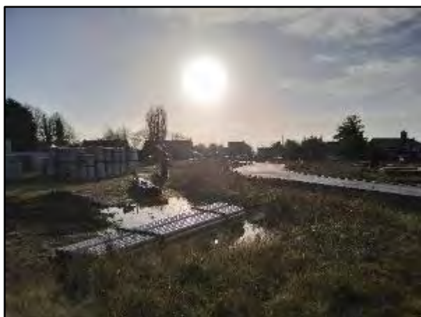
Photo 3 – A photo looking south towards the entrance to the site with the store and welfare yard to the left.
