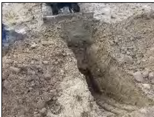
Photo 4 – A photo showing the excavation at TP1
