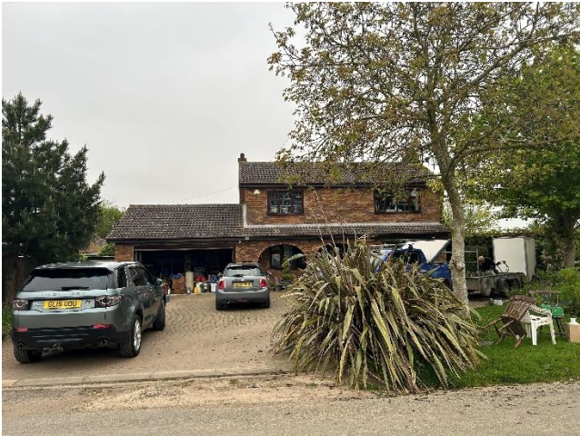
Front view showing existing garage and parking.
