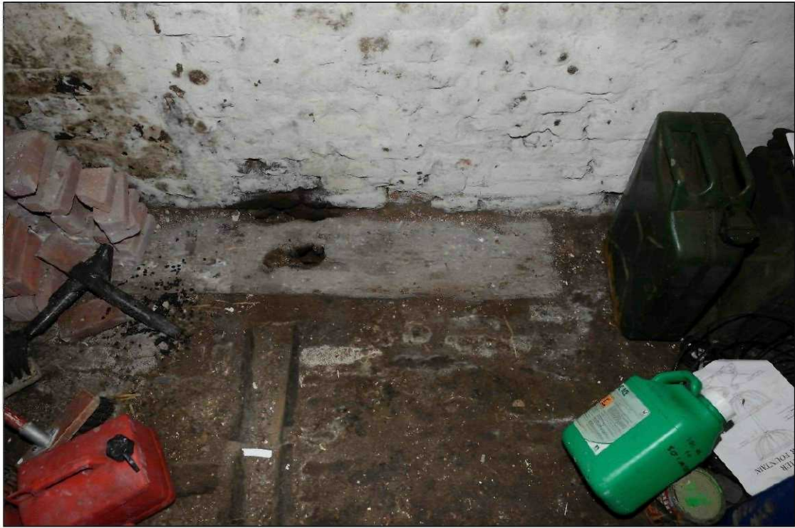
Plate 29: Building 1, reused timber incorporated into the stable floor, looking east
