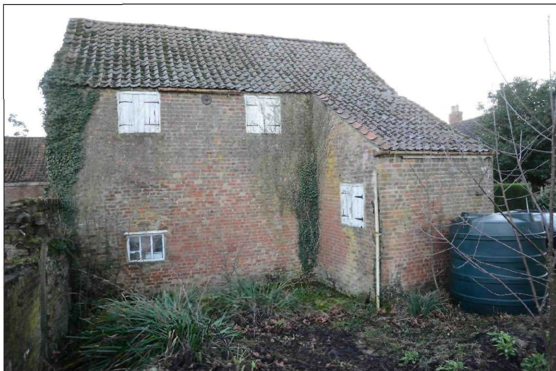
Plate 32: Building 2, north facing elevation, looking south
