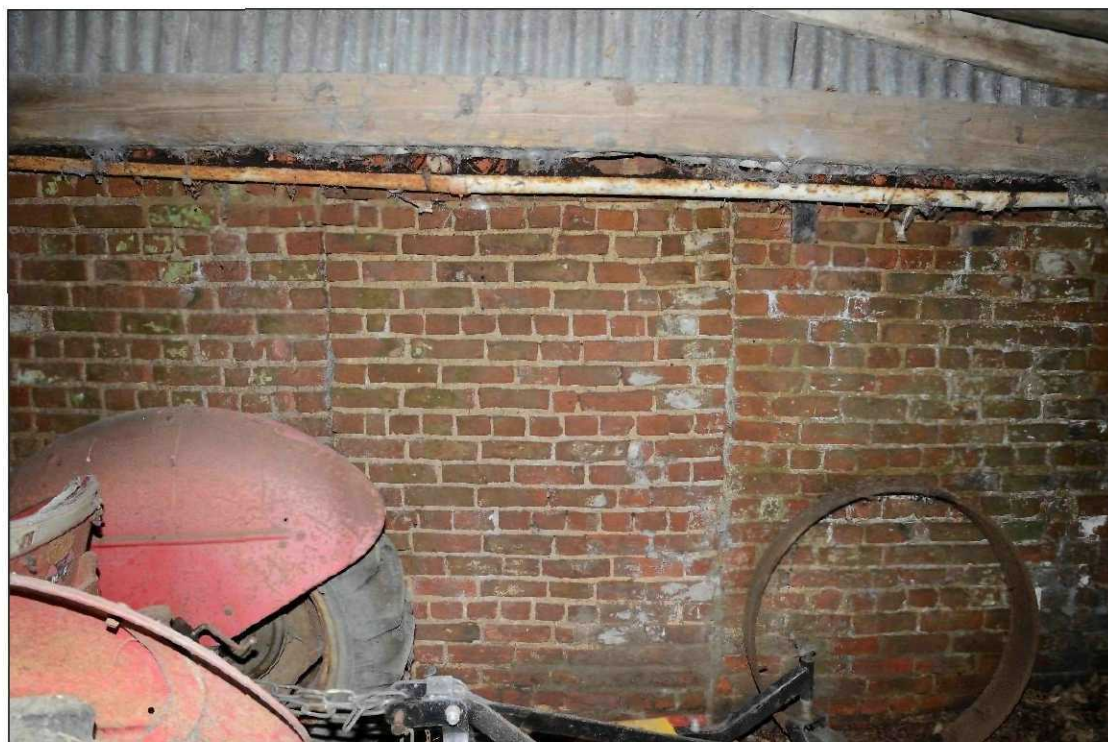
Plate 48: Building 3, blocked opening in the west wall, looking east
