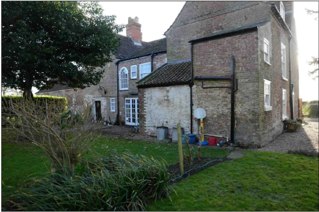
Plate 3: Austendike Hall, north facing elevation, looking southeast
