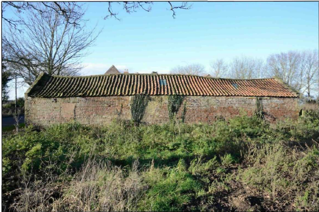
Plate 51: Building 3, east facing elevation, looking west
