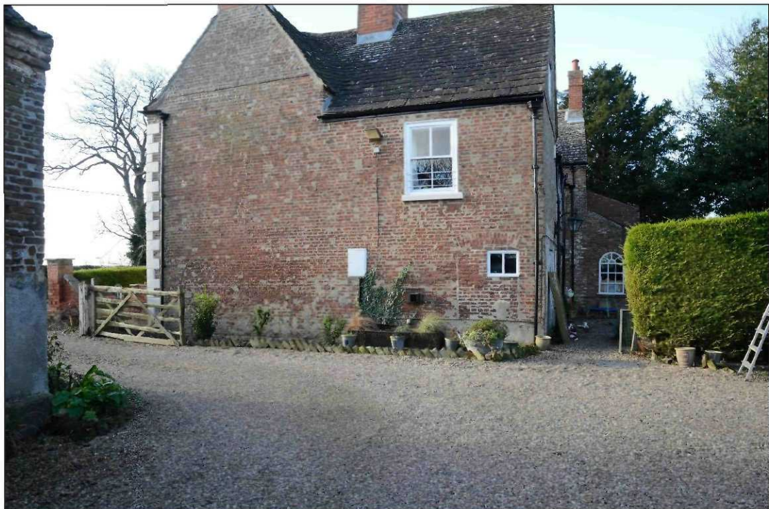
Plate 6: Austendike Hall, east facing elevation, looking west
