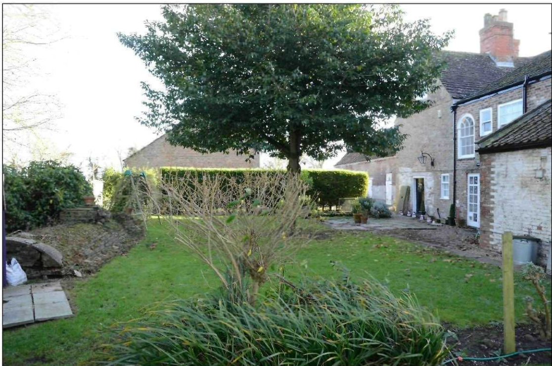
Plate 4: Austendike Hall, garden to the rear, looking southeast
