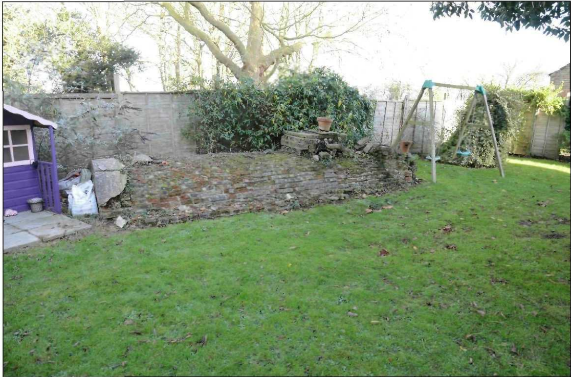
Plate 5: Probable coal cellar, looking northeast
