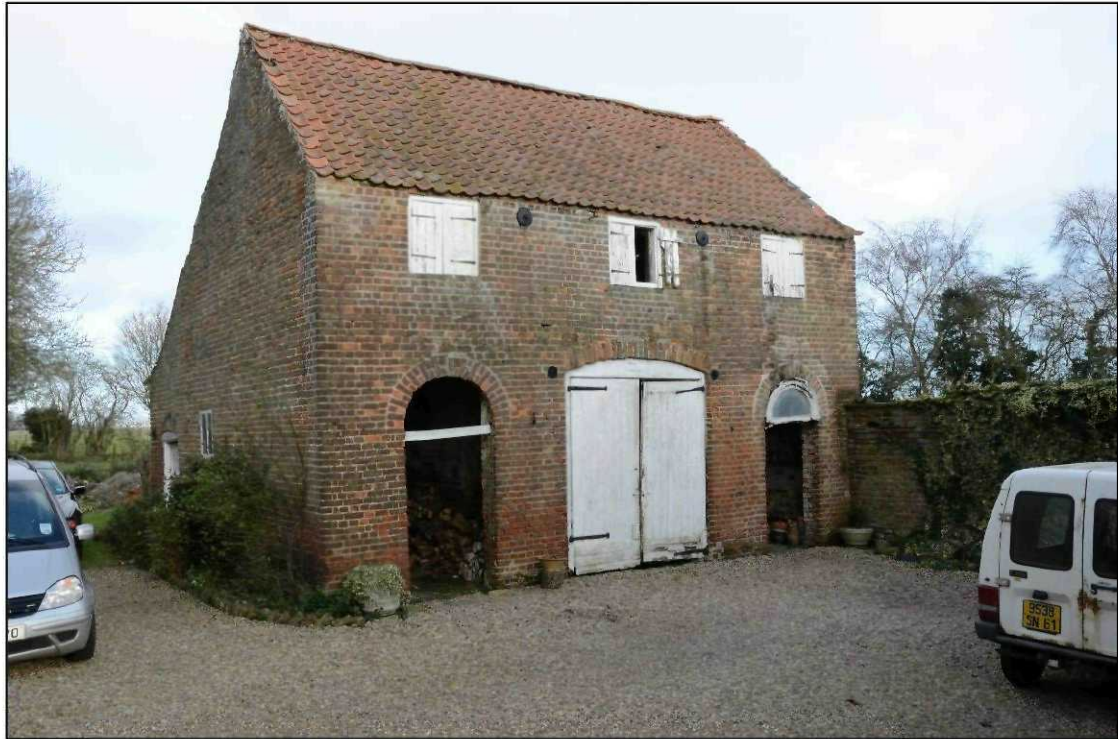
Plate 30: Building 2, south and west facing elevations, looking northeast
