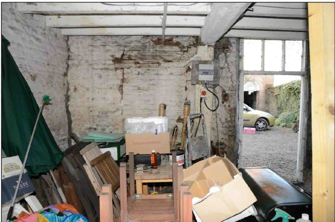
Plate 26: Building 1, blocked opening west of the stable door, looking north
