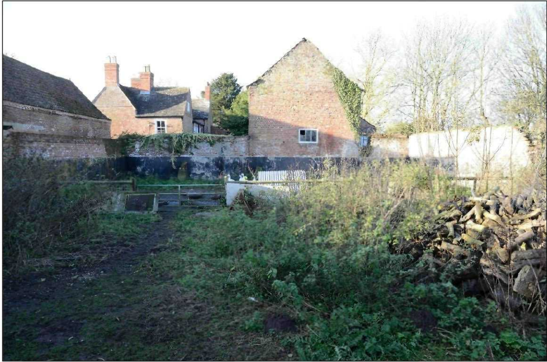
Plate 56: General view of yards and east facing elevation of Building 2, looking west
