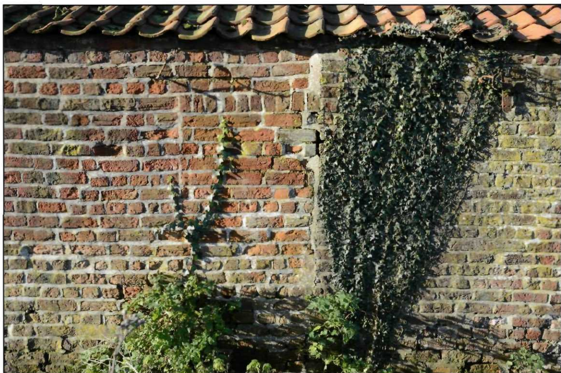
Plate 52: Building 3, east facing elevation, blocked opening and join, looking west
