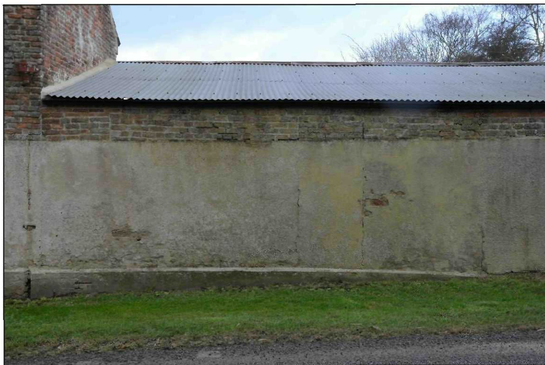
Plate 64: Wall between Buildings 1 and 3, looking north
