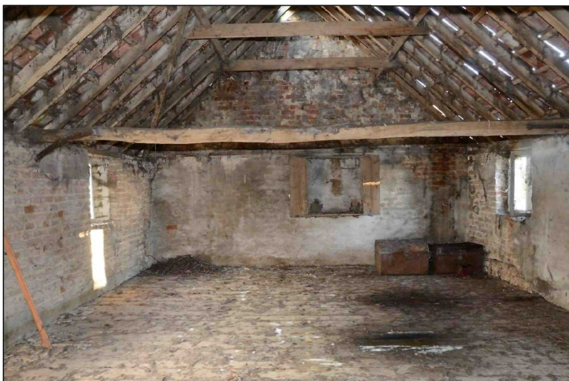
Plate 44: Building 2, east side of the 'granary', looking east
