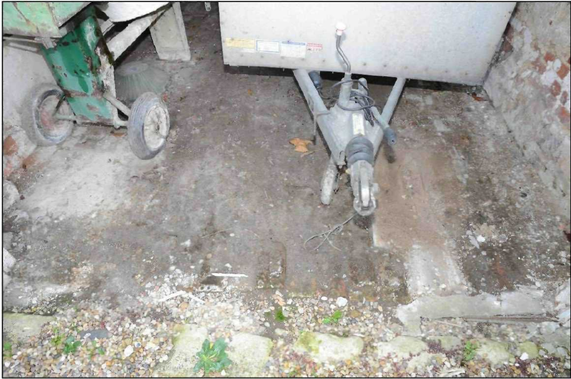
Plate 37: Building 2, 'coach/trap house' floor, looking north
