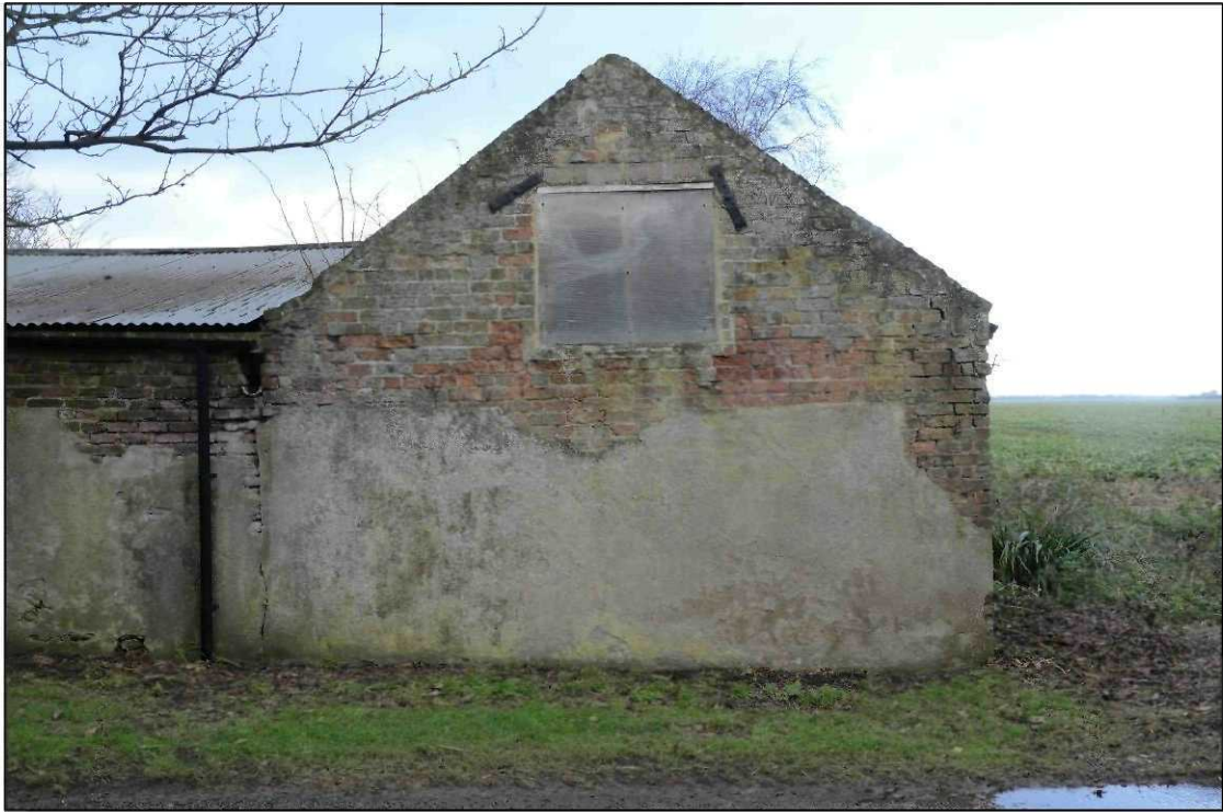
Plate 53: Building 3, south facing elevation, looking north
