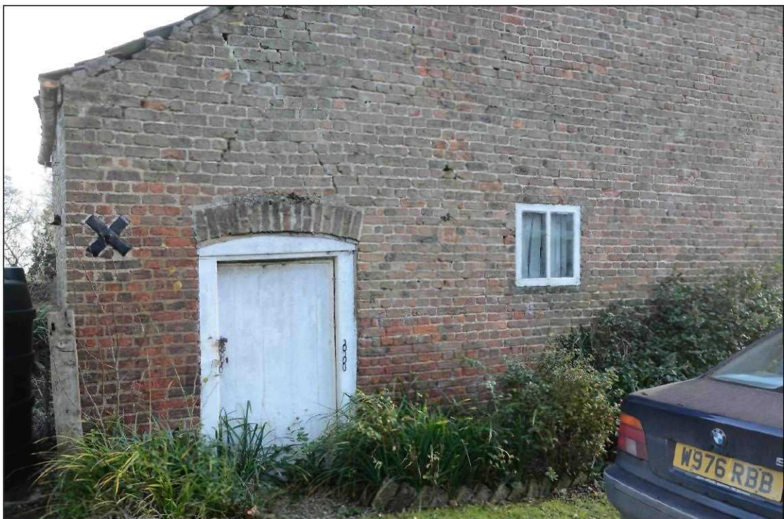
Plate 31: Building 2, door and window in the west facing elevation, looking east
