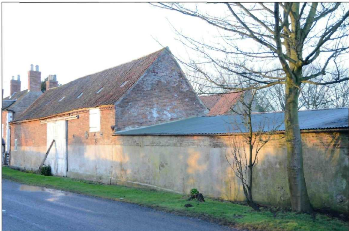
Plate 12: Building 1, south and east facing elevations, looking northwest
