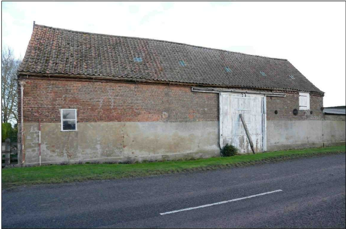
Plate 7: Building 1, south facing elevation, looking northeast
