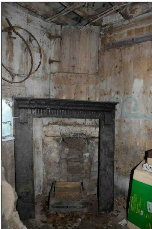
Plate 34: Building 2, fireplace in the 'tack room', looking northeast
