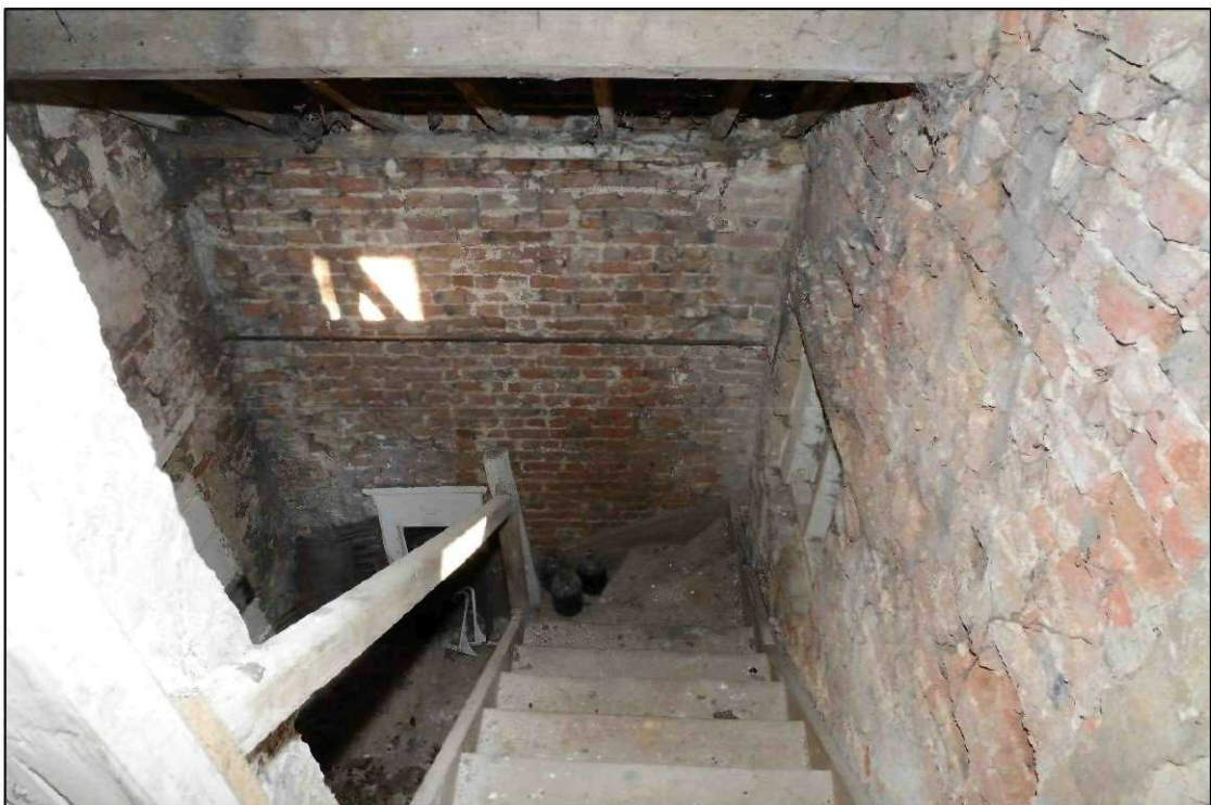
Plate 40: Building 2, covered entrance to 'granary', looking north
