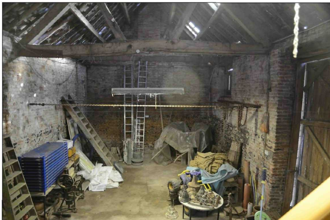
Plate 13: Building 1, threshing barn interior, looking east
