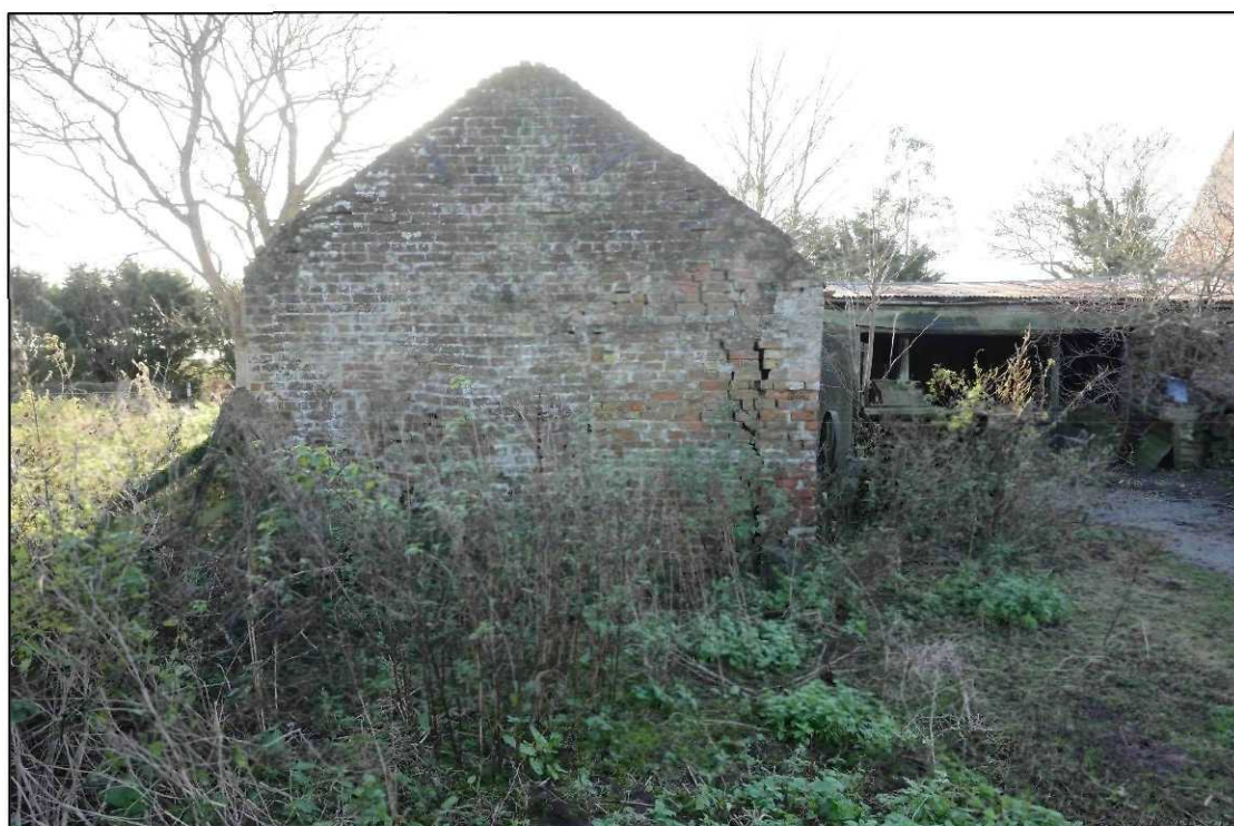
Plate 50: Building 3, north facing elevation, looking south
