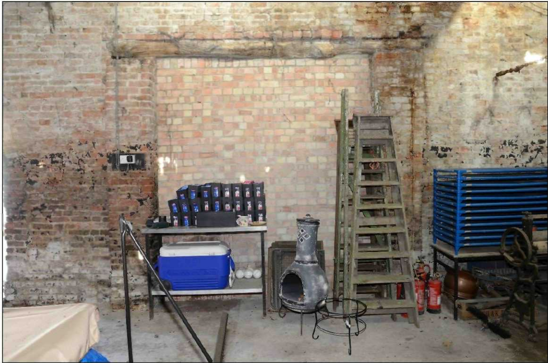
Plate 17: Building 1, interior of north door, looking north
