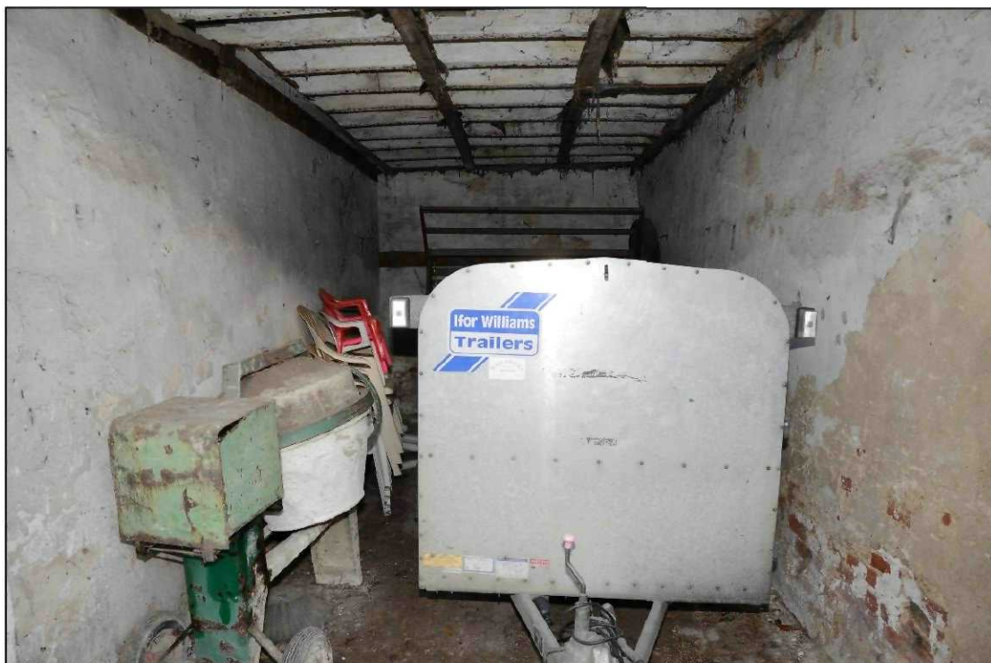
Plate 36: Building 2, 'coach/trap house' interior, looking north
