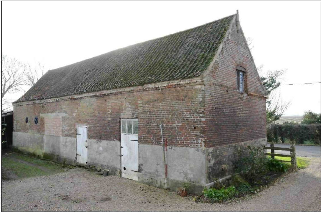
Plate 9: Building 1: west and north facing elevations, looking southeast
