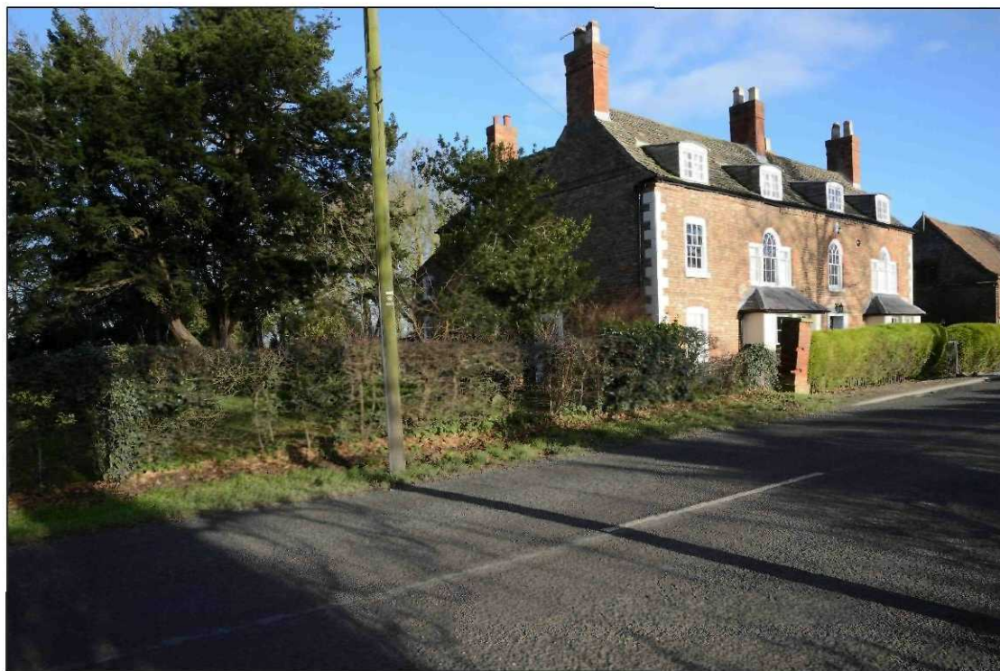
Plate 1: Austendike Hall, south facing elevation, looking northeast
