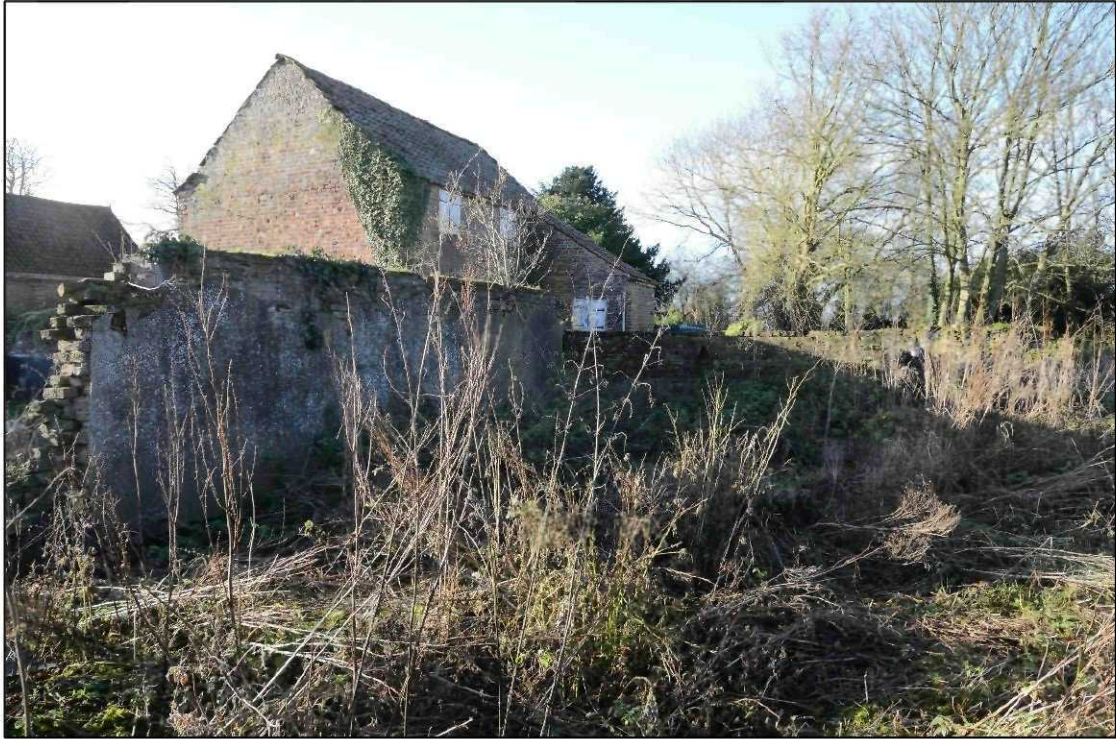
Plate 60: Building 4, south (to left) and west (to right) walls, looking west
