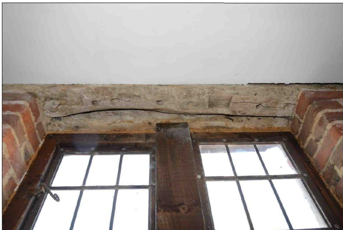
Plate 22: Building 1, lintel (reused) over the 'hayloft' window, looking west
