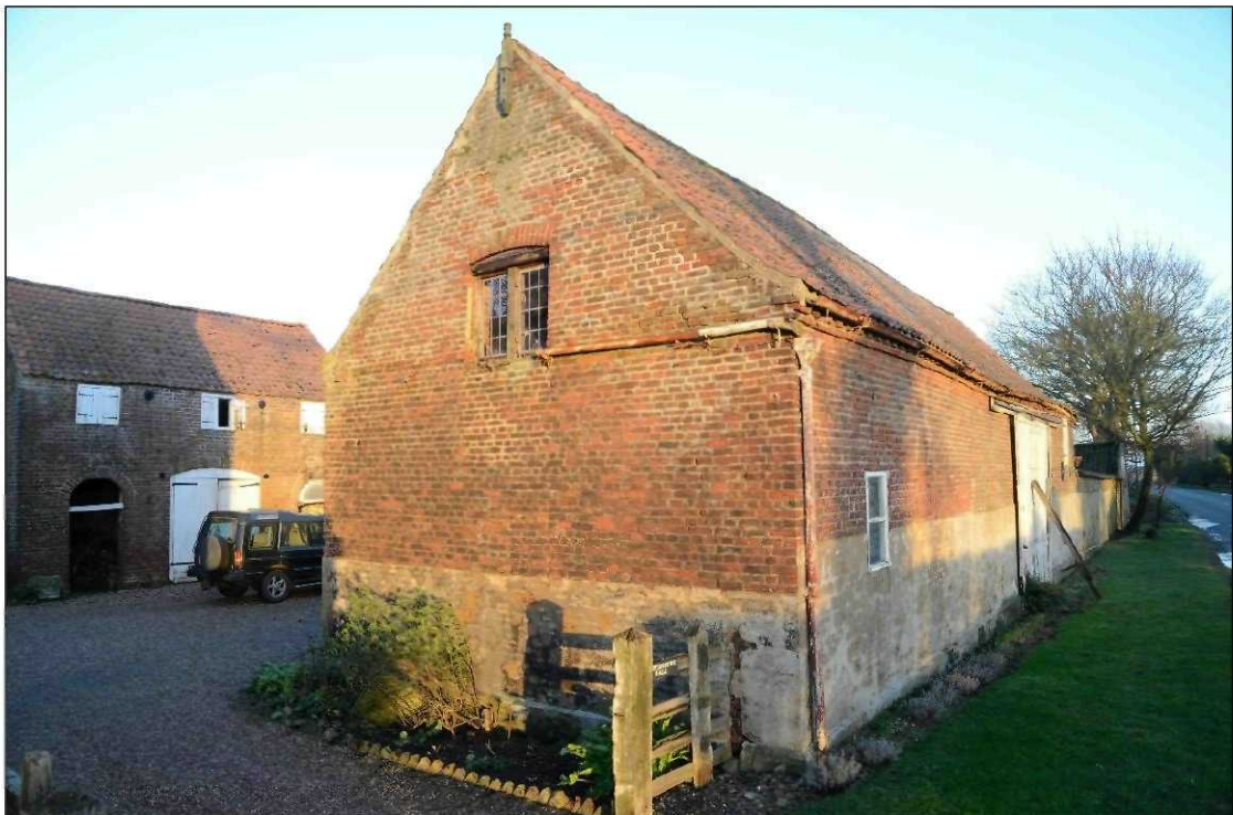
Plate 8: Building 1, west and south facing elevations, looking east
