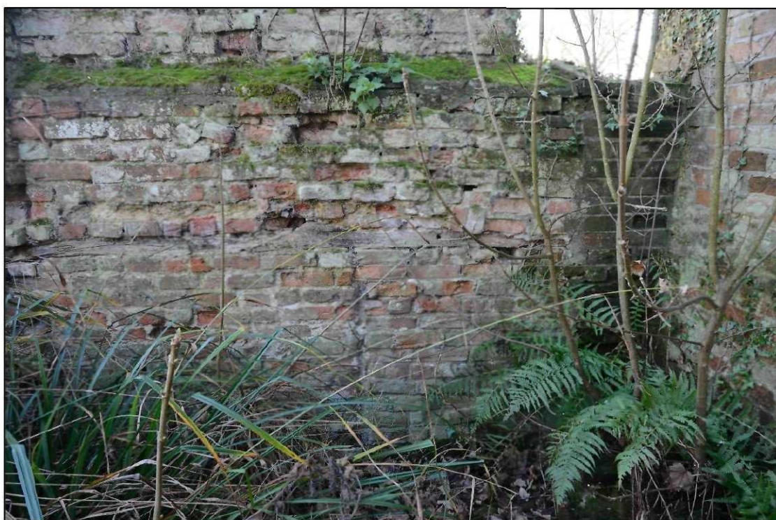
Plate 63: Blocked opening to the probable pig sty and/or hen house (see Plate 62), looking east
