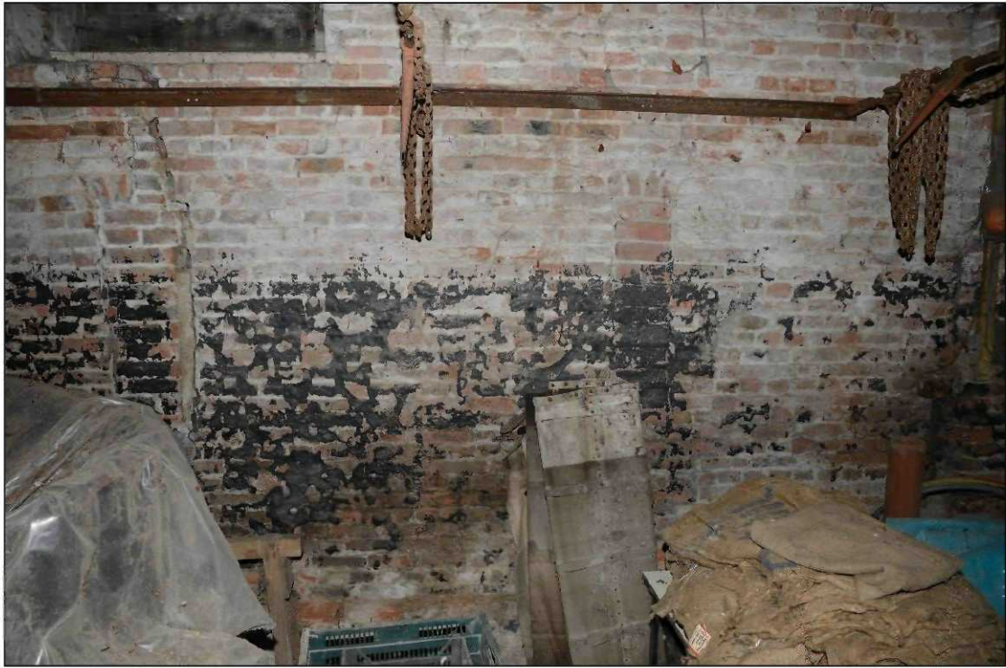
Plate 19: Building 1, pair of blocked ventilation slots, looking south
