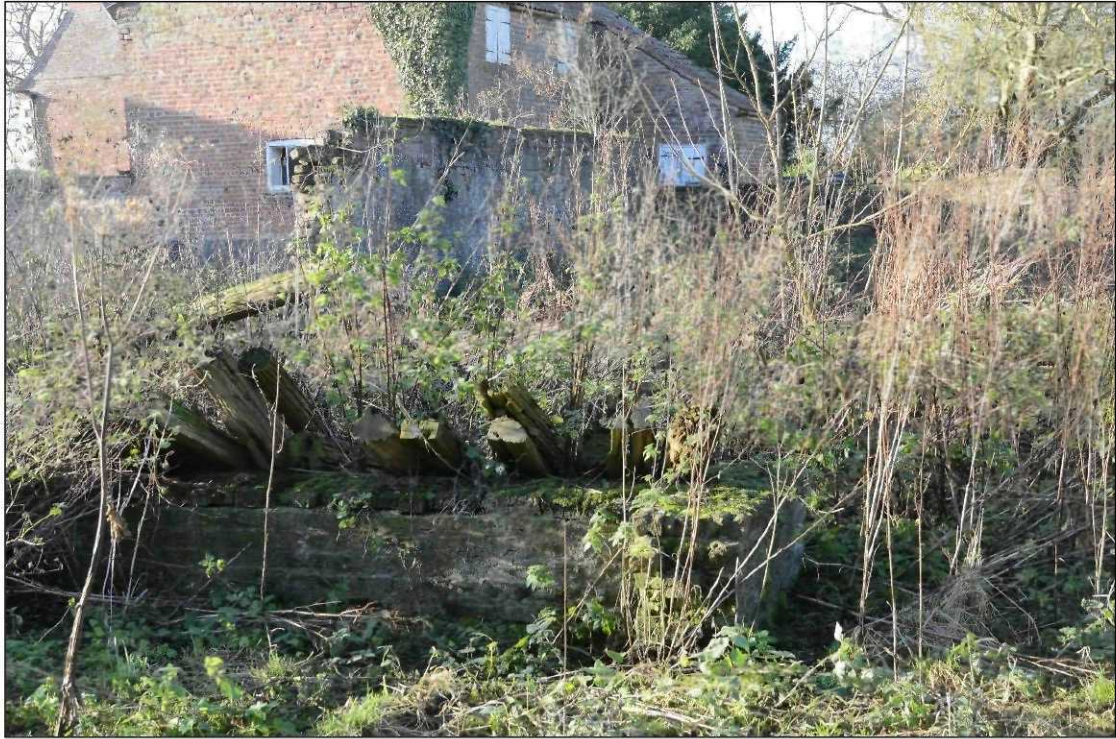
Plate 58: Building 4, east (in foreground), south (to left) and west walls, looking west
