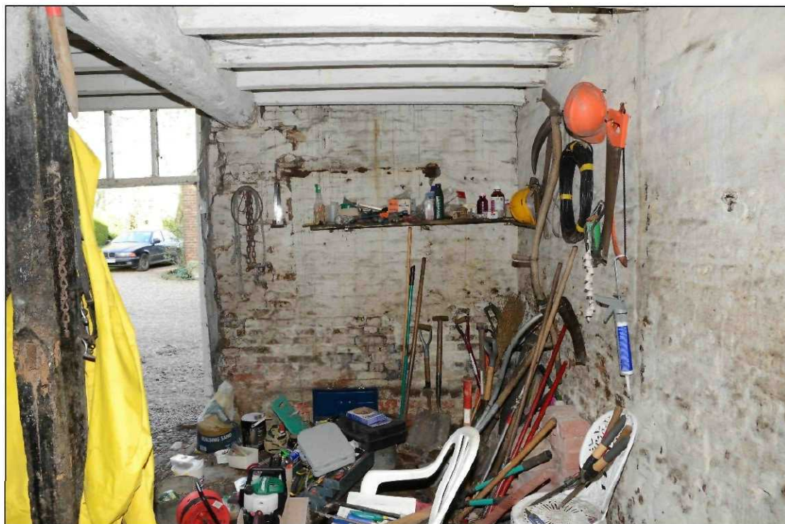
Plate 27: Building 1, blocked opening east of the stable door, looking north
