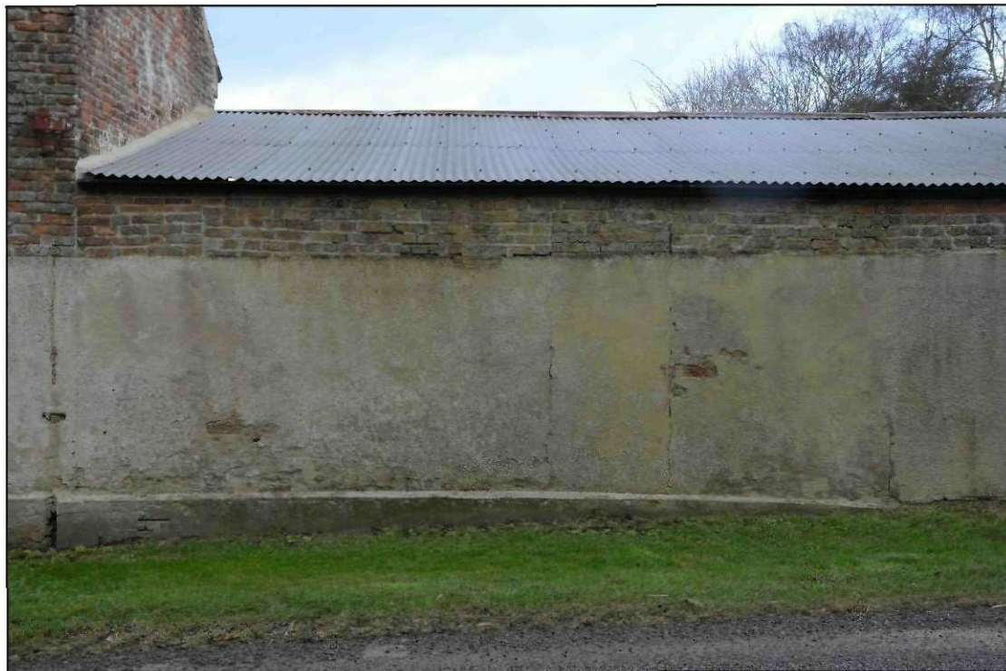
Plate 64: Wall between Buildings 1 and 3, looking north
