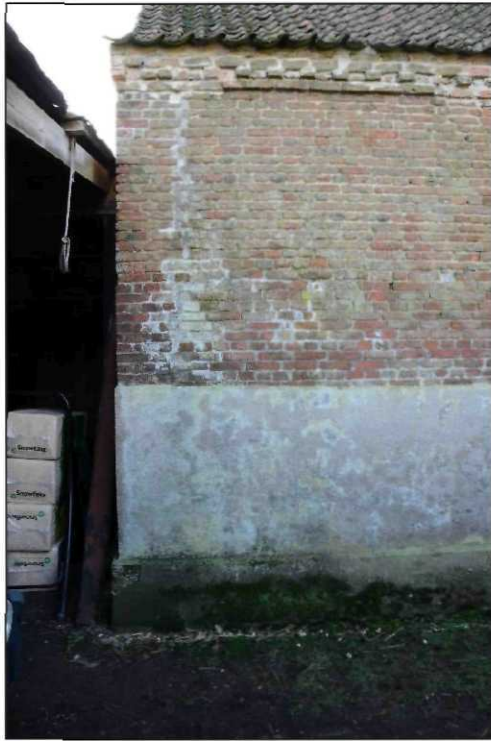
Plate 11: Building 1, north facing elevation (eastern end), looking c. south
