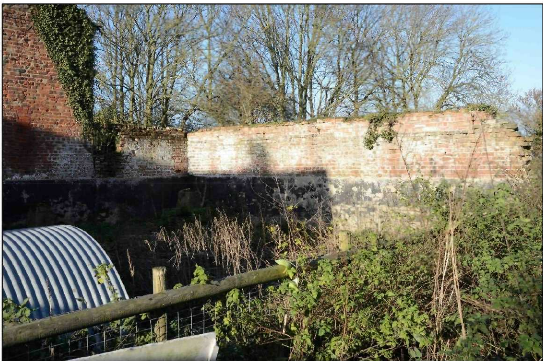
Plate 57: Building 4, south wall, looking northwest
