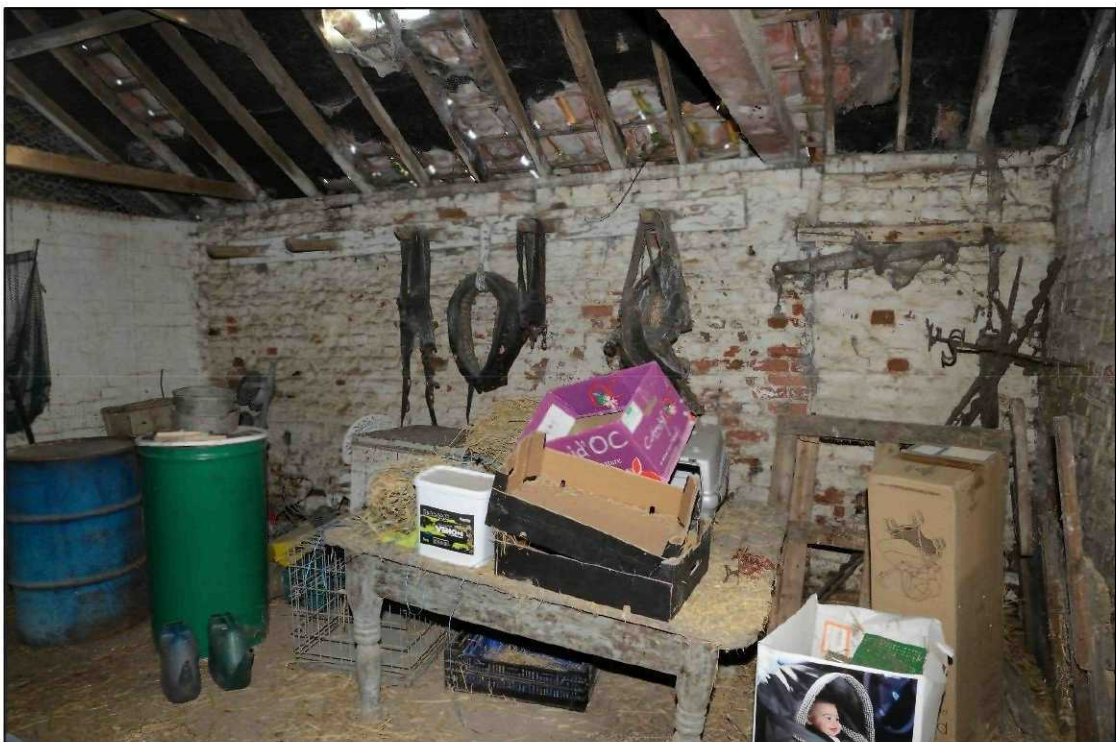
Plate 54: Building 3, interior of the central unit, looking east
