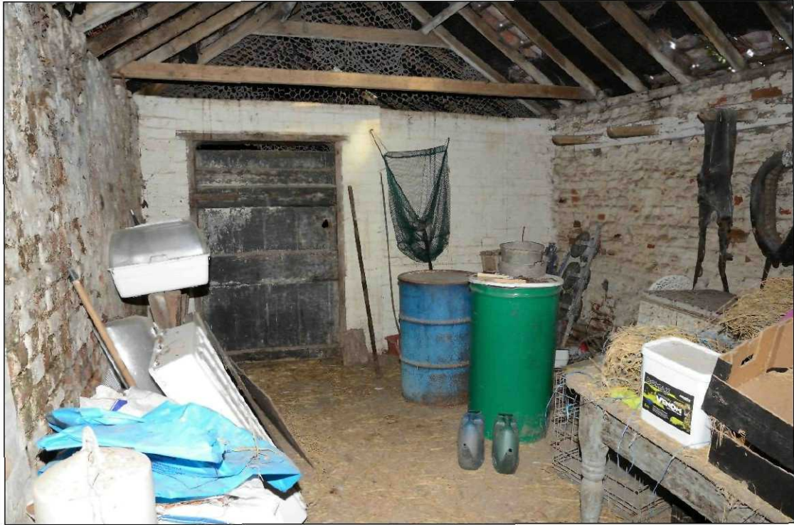
Plate 55: Building 3, interior of the central unit, looking c. north
