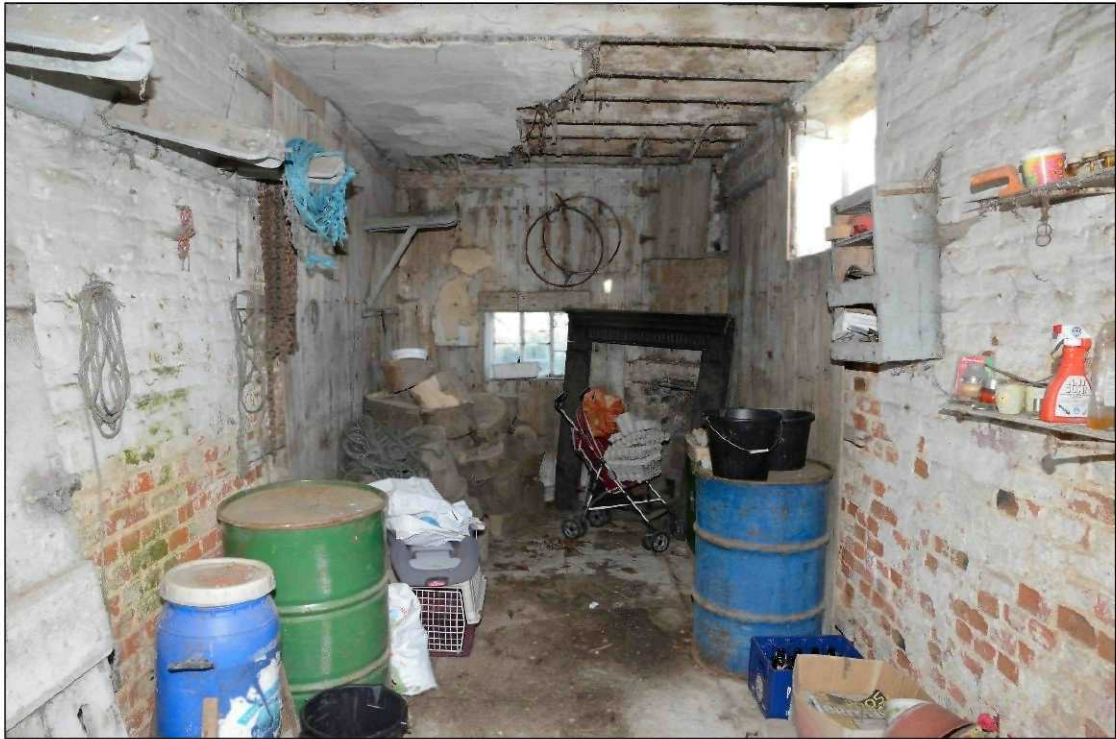
Plate 33: Building 2, 'tack room' interior, looking north
