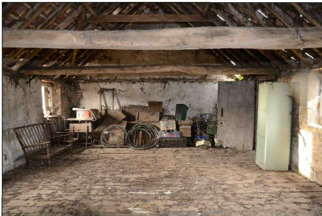
Plate 43: Building 2, west side of the 'granary', looking west
