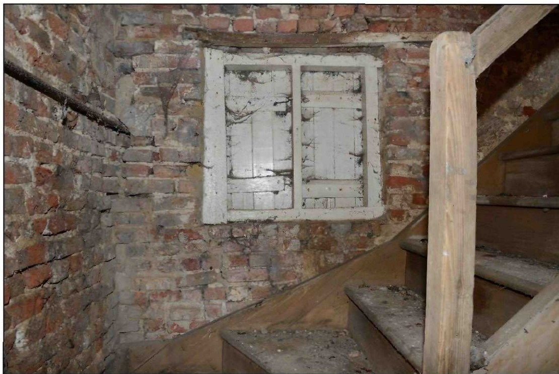
Plate 41: Building 2, window in covered entrance, looking east
