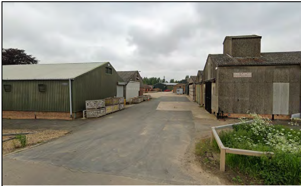
Existing Buildings from High Road
