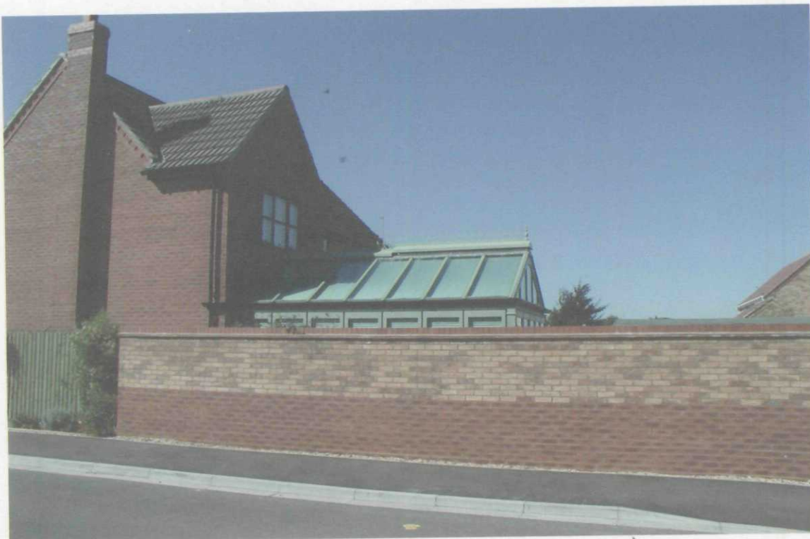
no. 19. (to rear of no. 1 Braybrooks)
